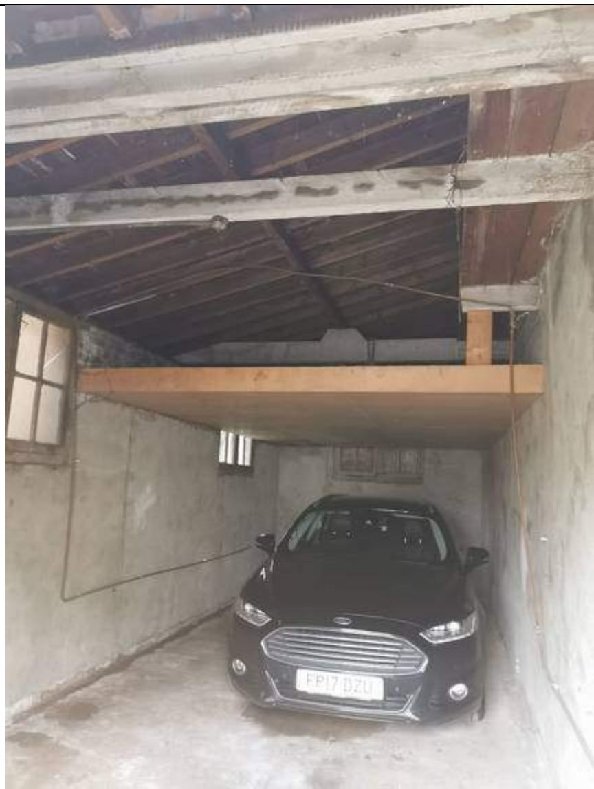
Plate 3 – internal area of garage (third party supply)
