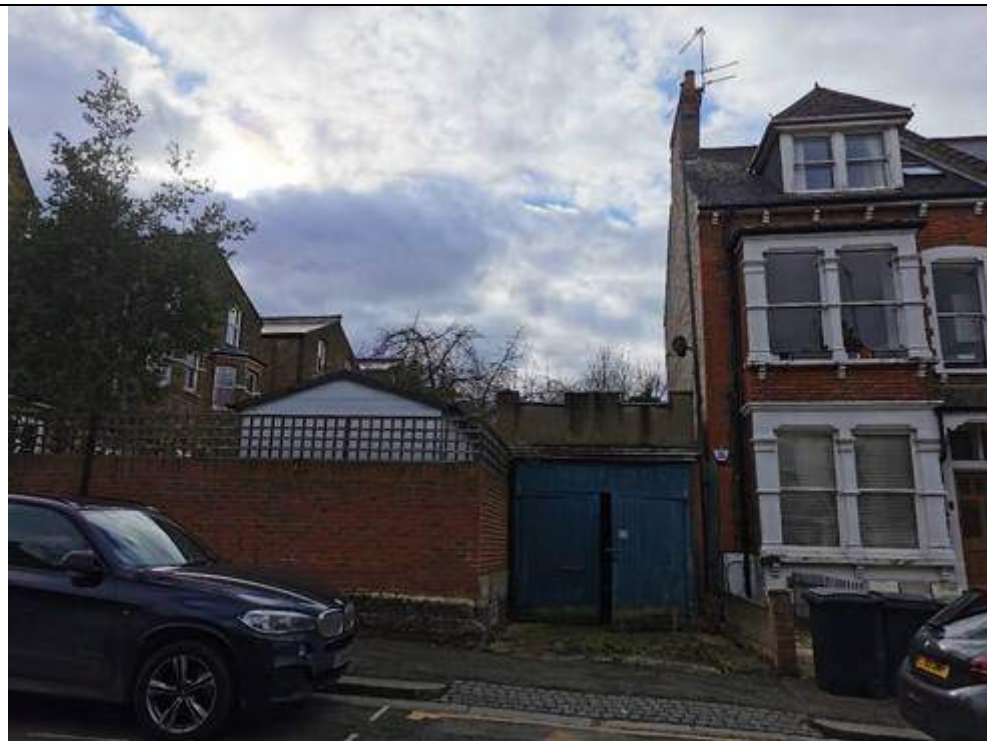
Plate 1 – front of garage building
