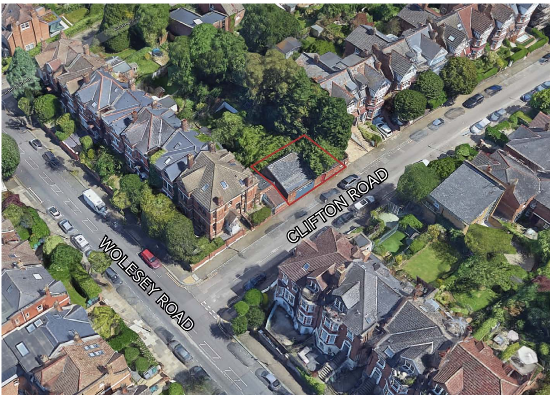
Fig.1 Aerial view of site
