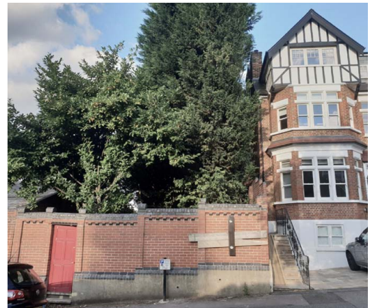
Fig.4 Existing brick wall and over grown hedge on site
