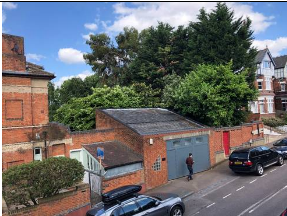
Photo 1 – View of site from Clifton Rd
