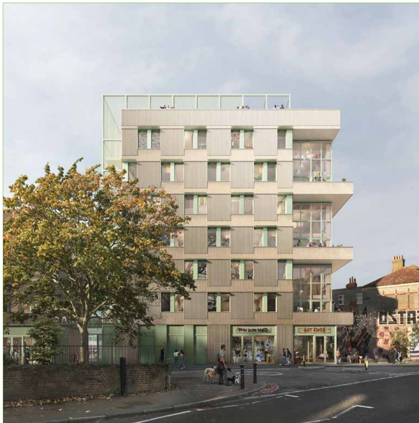
Image 5.2 - Marking the gateway to the warehouse district
