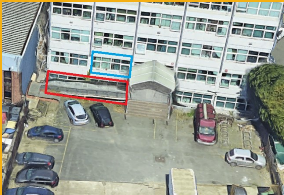
Windows with noticeable overshadowing in Cara house do not meet criteria in current conditions.
