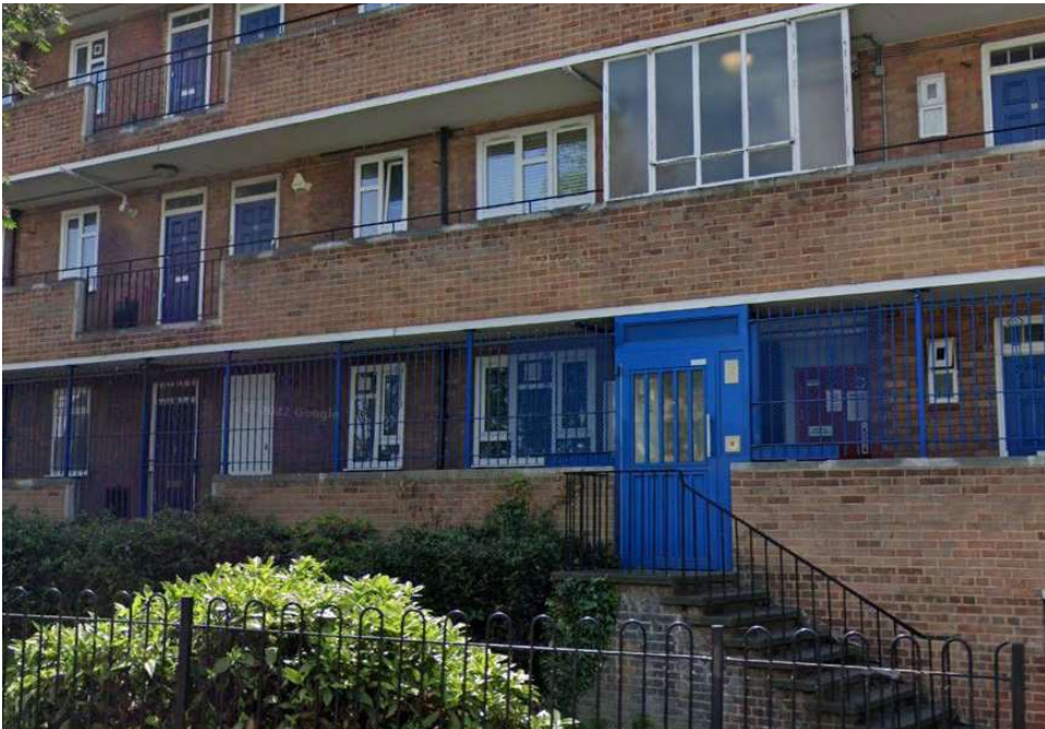
2. Vivian House Entrance off Eade road*
