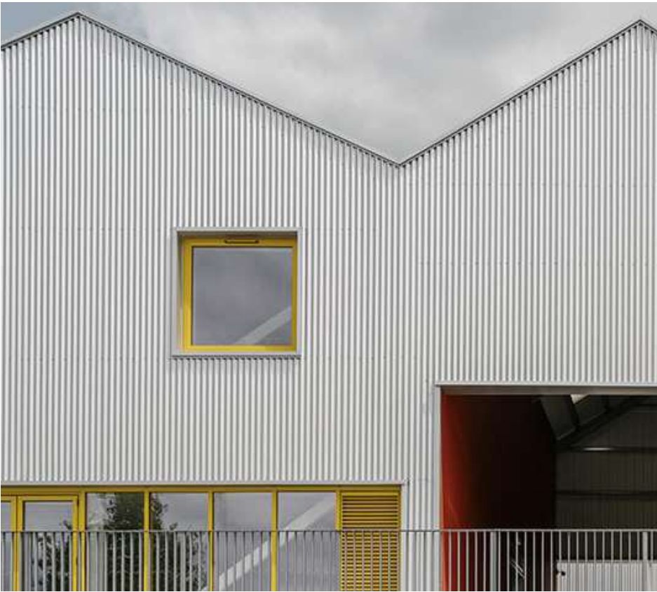
Corrugated sheet materials Simple corrugated materials offset with colour gives the architecture greater depth and interest
