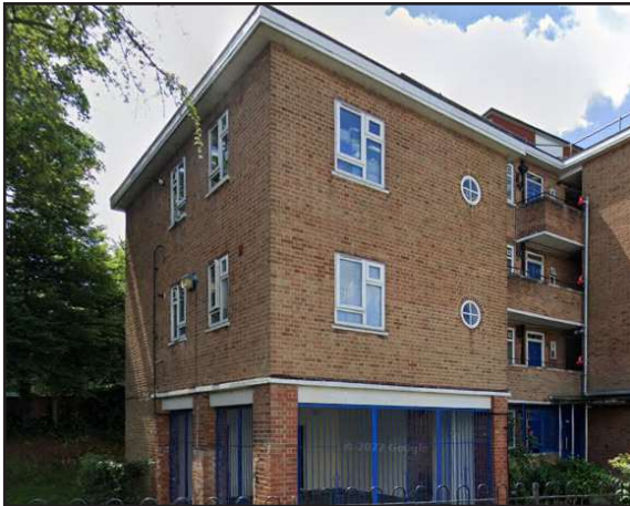
Vivian House, Eade Road
