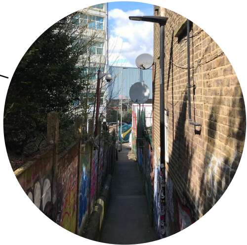
The existing alley is faced with totally blank facades with no overlooking and with no means of escape, making the space feel intimidating. The level of disrepair adds to this impression.
