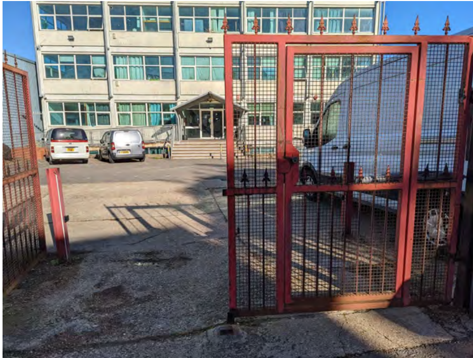
Image 1: Main site entrance to the south of the site. Opposite Cara House.
