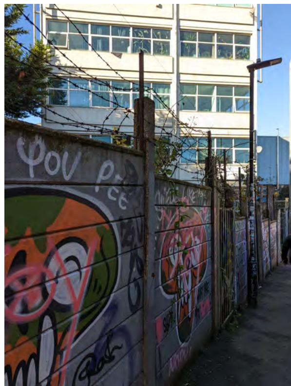
Image 12: Passage way – eastern side of the site.
