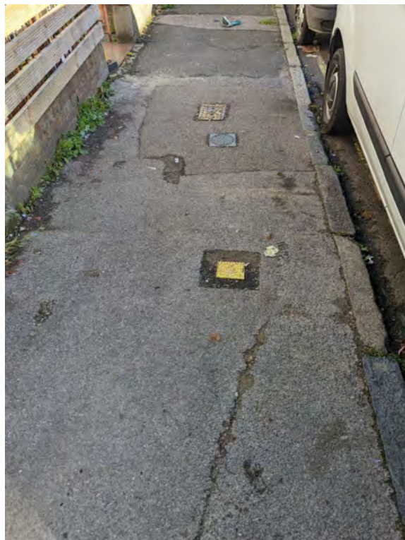
Image 8: Thames Water monitoring wells located on site at the end of Tewksbury Road.
