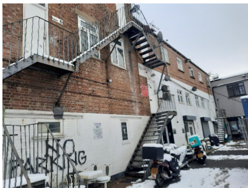
Plate 3: Rear of Building B11, next to construction area.
