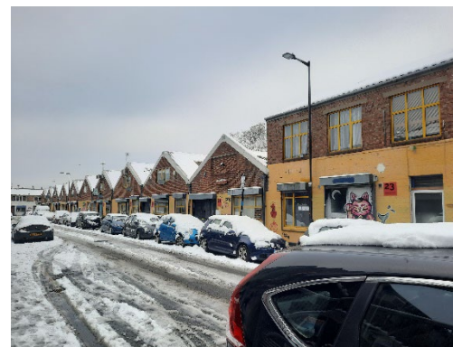
Plate 4: Building B10, south side.
