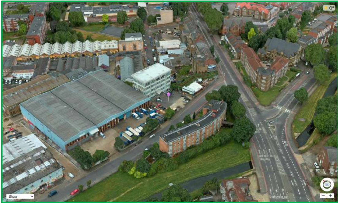
The Site – Viewed From South West
