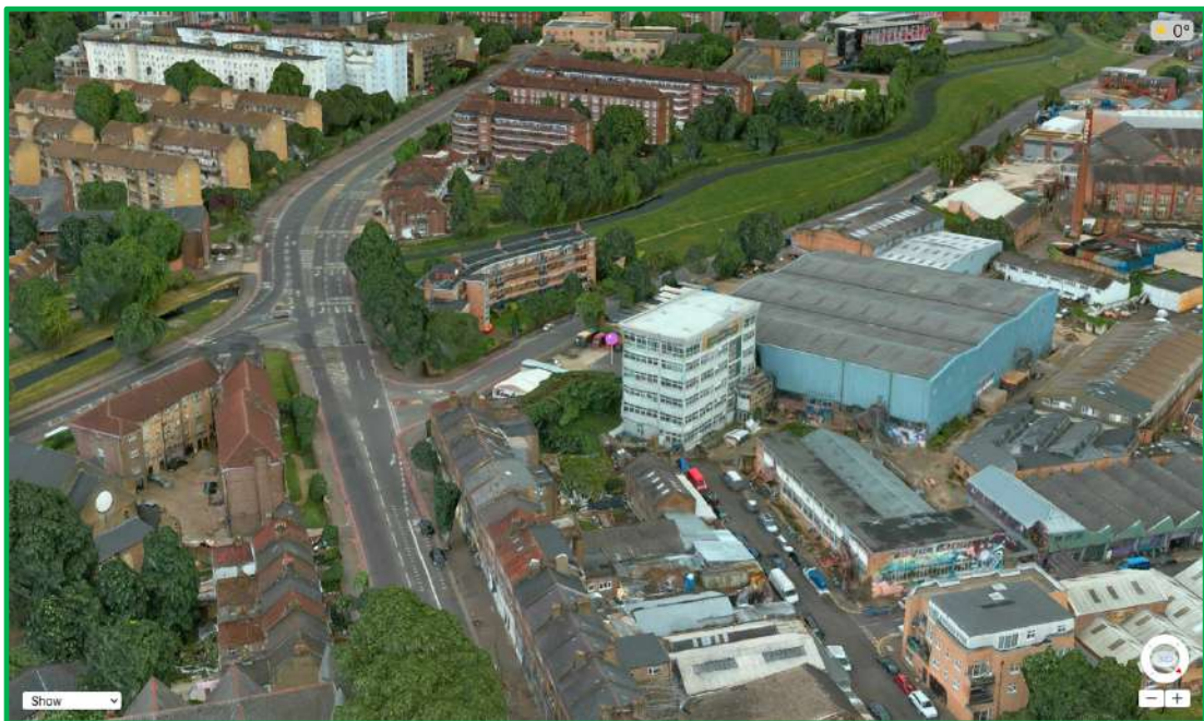
The Site – Viewed From North East
