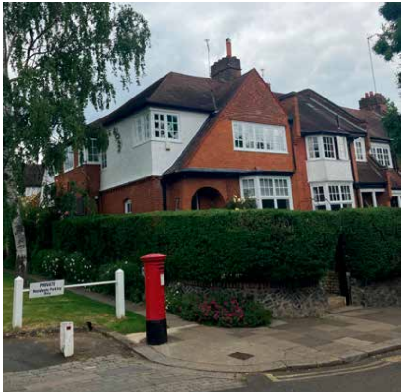
Fig. 4.7: Special end of terrace at junction of Etheldene Avenue and Rookfield Avenue.
