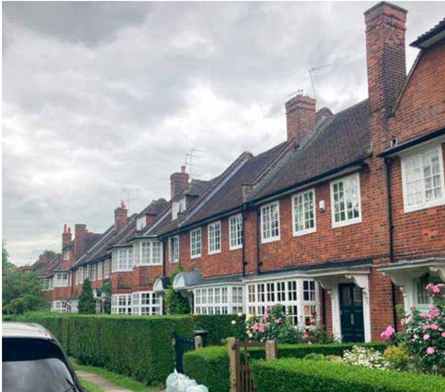
Fig. 4.13: Cascade Avenue looking north.
