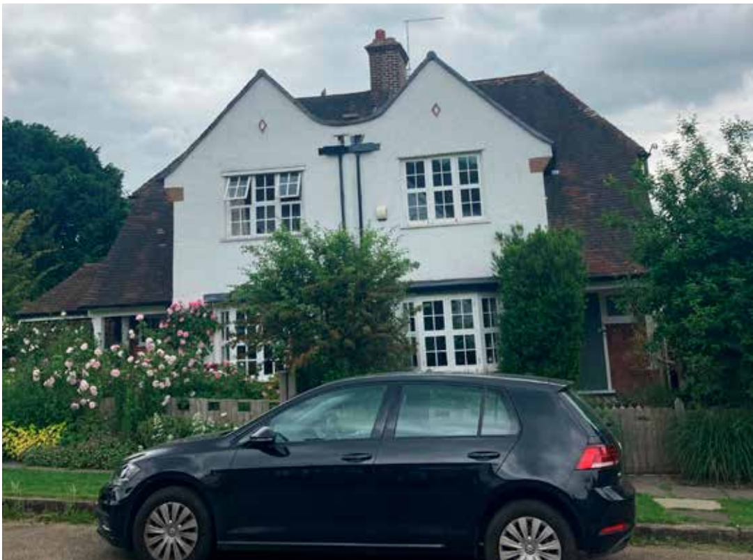
Fig. 4.6: Double gabled house.
