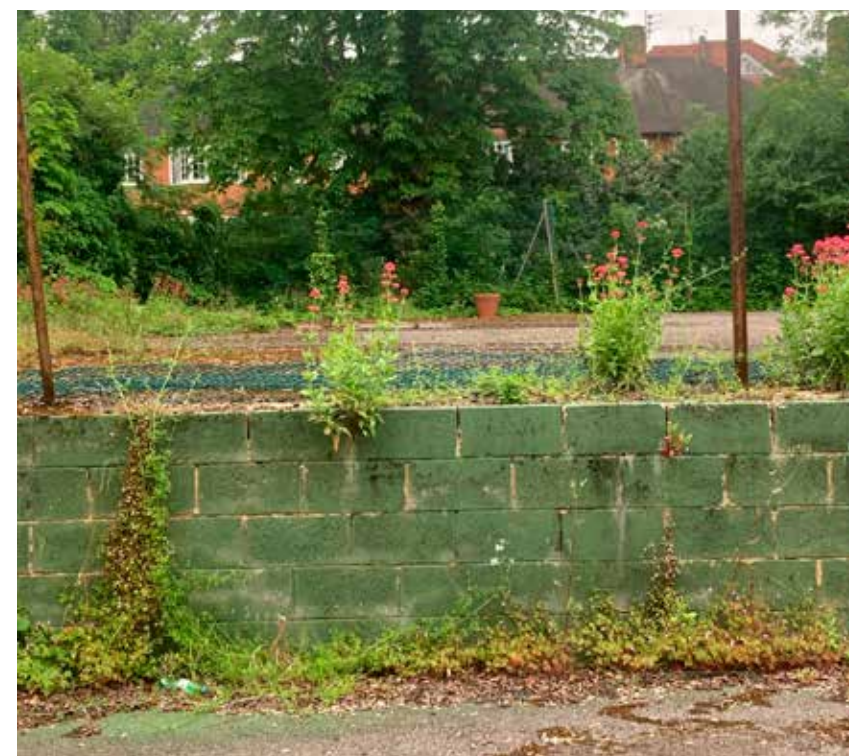
Fig. 2.13: The retaining block wall.
