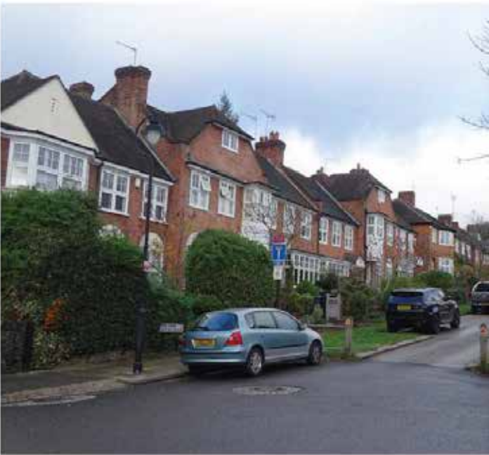
The Chine - View from the South
