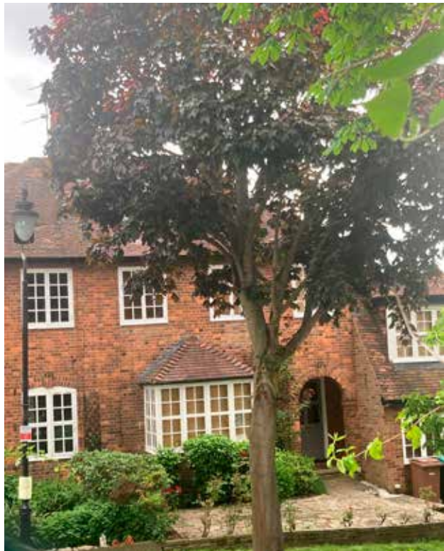
Fig. 4.15: Cascade Avenue - detail.
