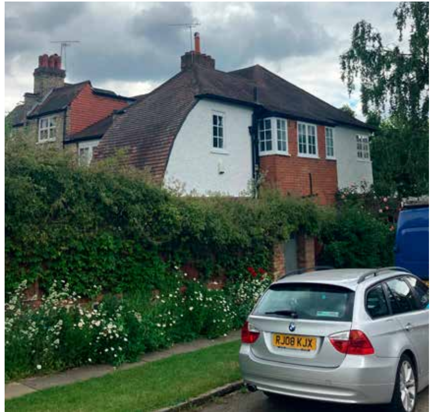
Fig. 4.8: The west side of the same house with an articulated elevation in varied materials and its idiosyncratic curved roof.
