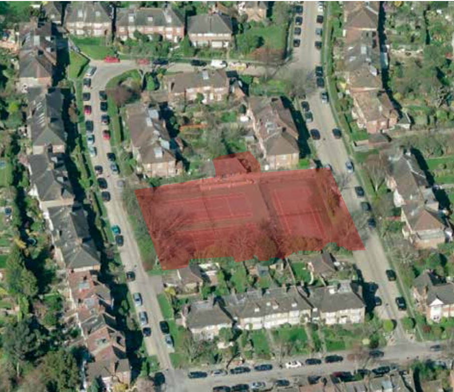
Fig. 1.1: Aerial view of the site with its approximate extent marked in red (Bing, 2022).
