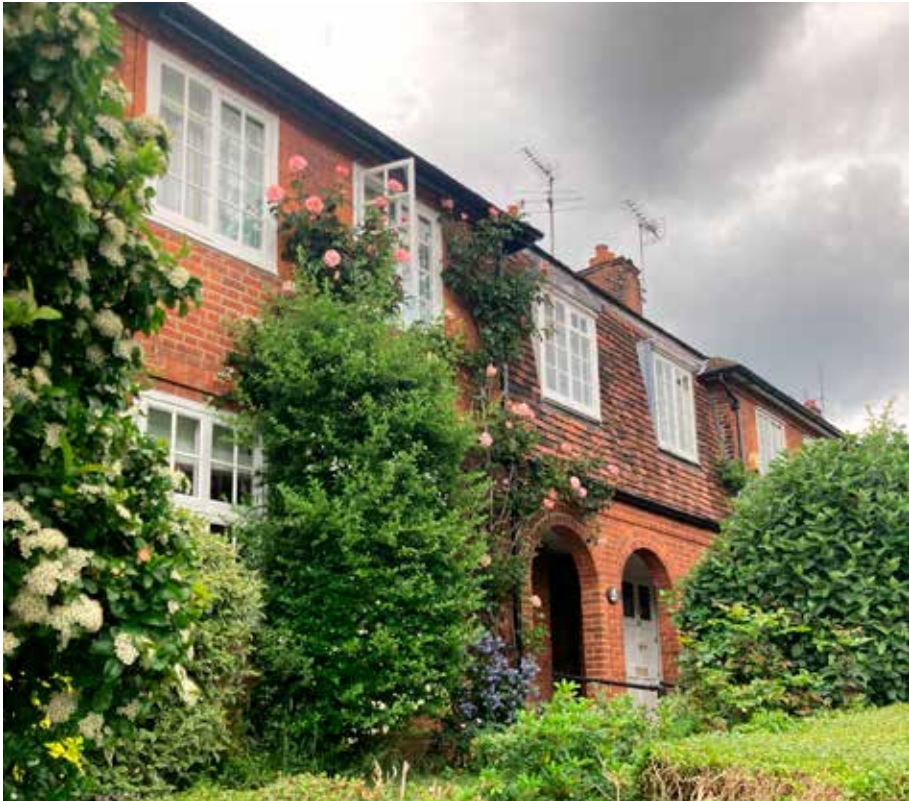
Fig. 4.12: The Chine west side.
