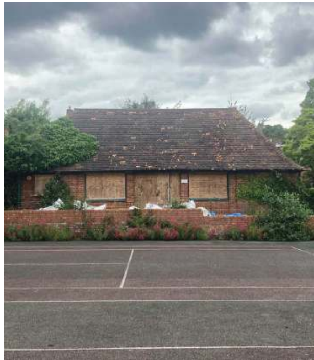
Figure 5.2 The pavilion building to the north of the Site (Source: Adam Architecture)
