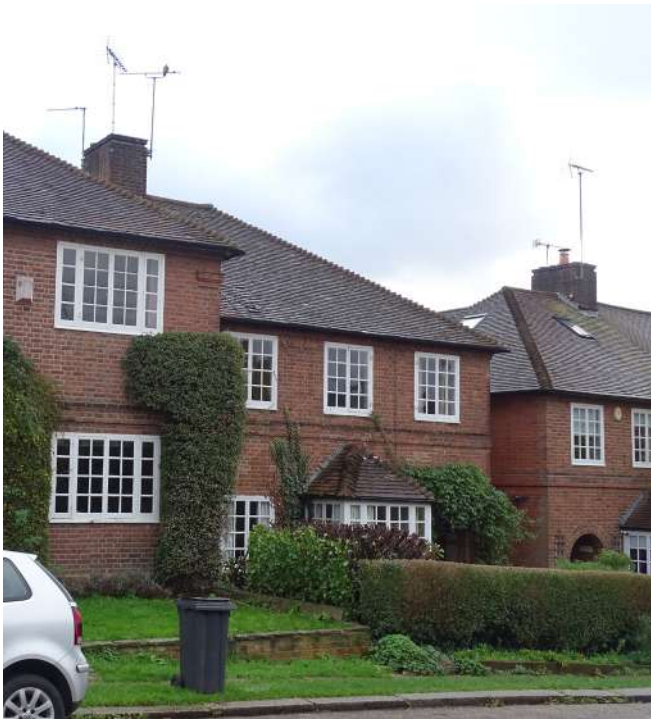
Cascade Avenue - North
