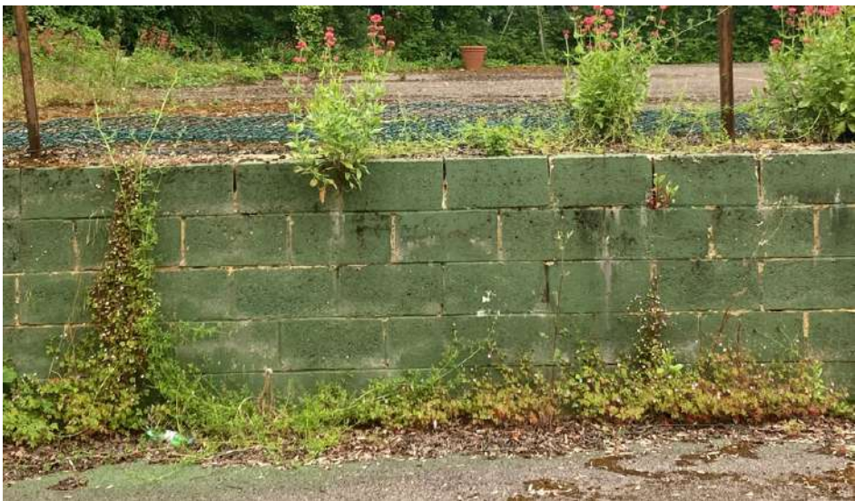
The retaining block wall
