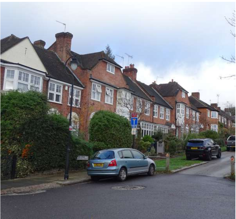
The Chine - View from the South
