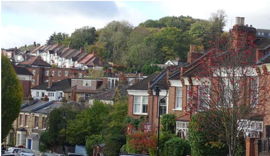
View of the roofscape from St James's Ln
