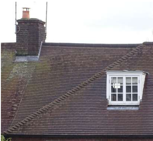
Brown plain clay tiles and simple dormer windows
