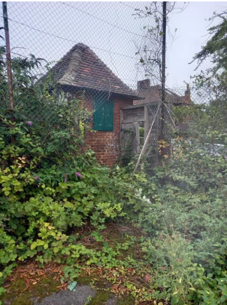
Site Entrance, looking north-east.
