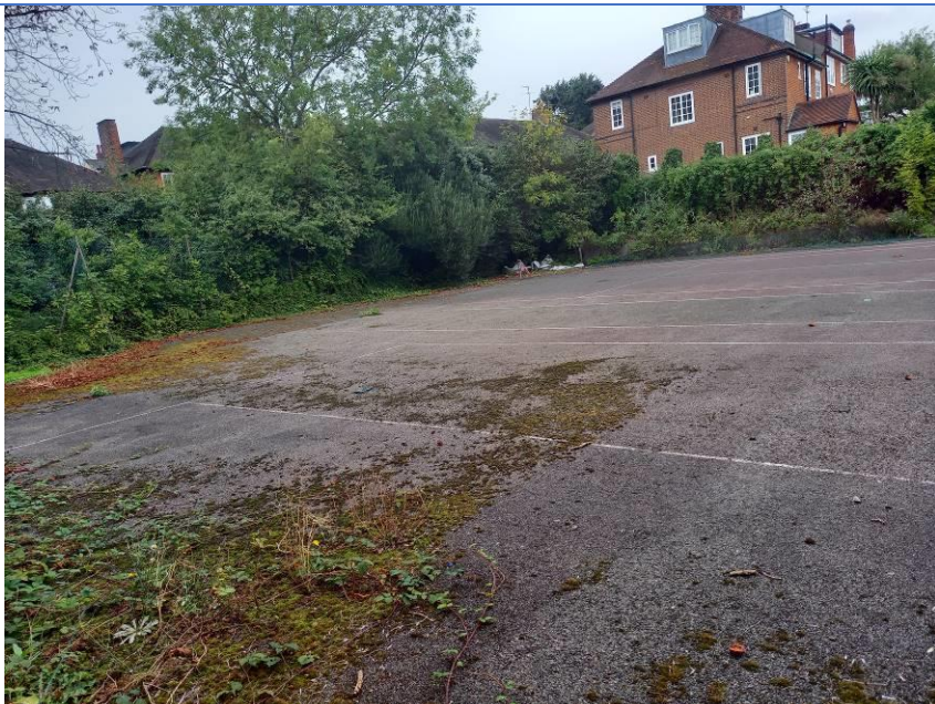
Westernmost tennis courts looking north-west, from south-western corner
