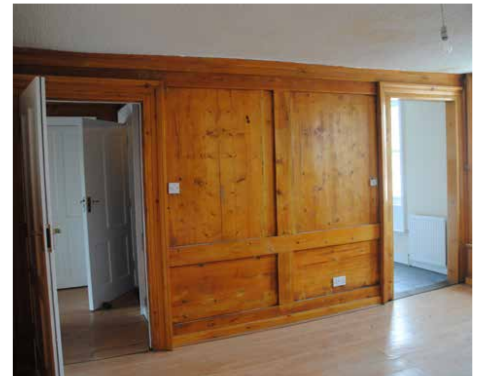
FIGURE 39. Overall View Looking South
