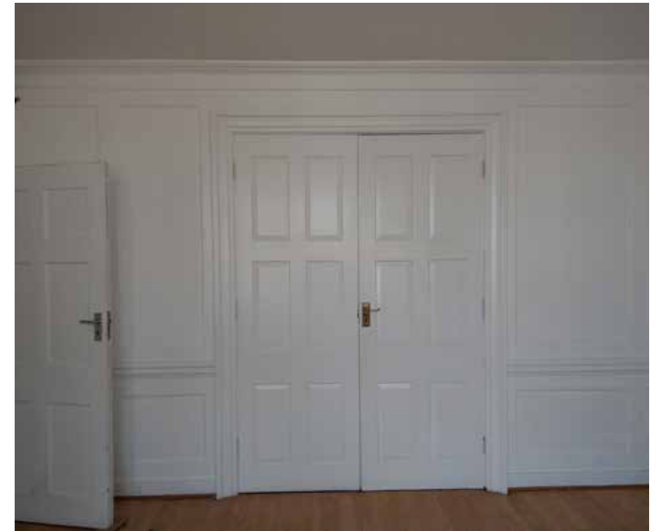
FIGURE 4. Overall West Elevation
