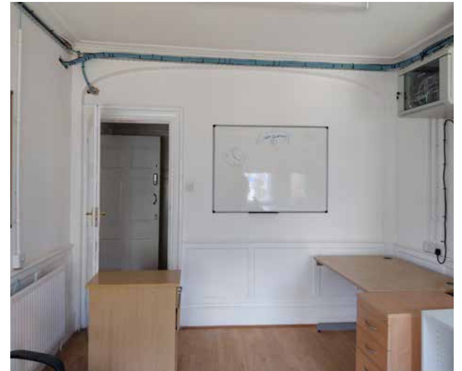
FIGURE 15. Existing Panelling and Ceiling Cornice
