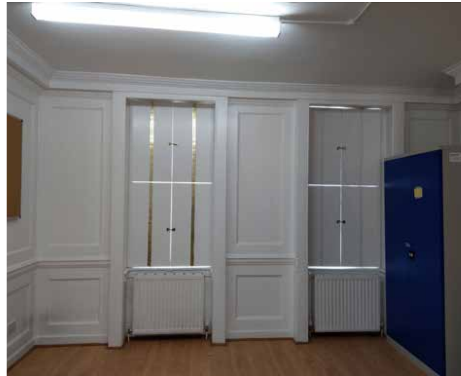
FIGURE 6. Overall West Elevation
