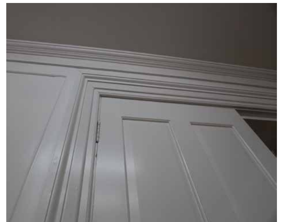
FIGURE 3. Existing Architrave and Ceiling Cornice
