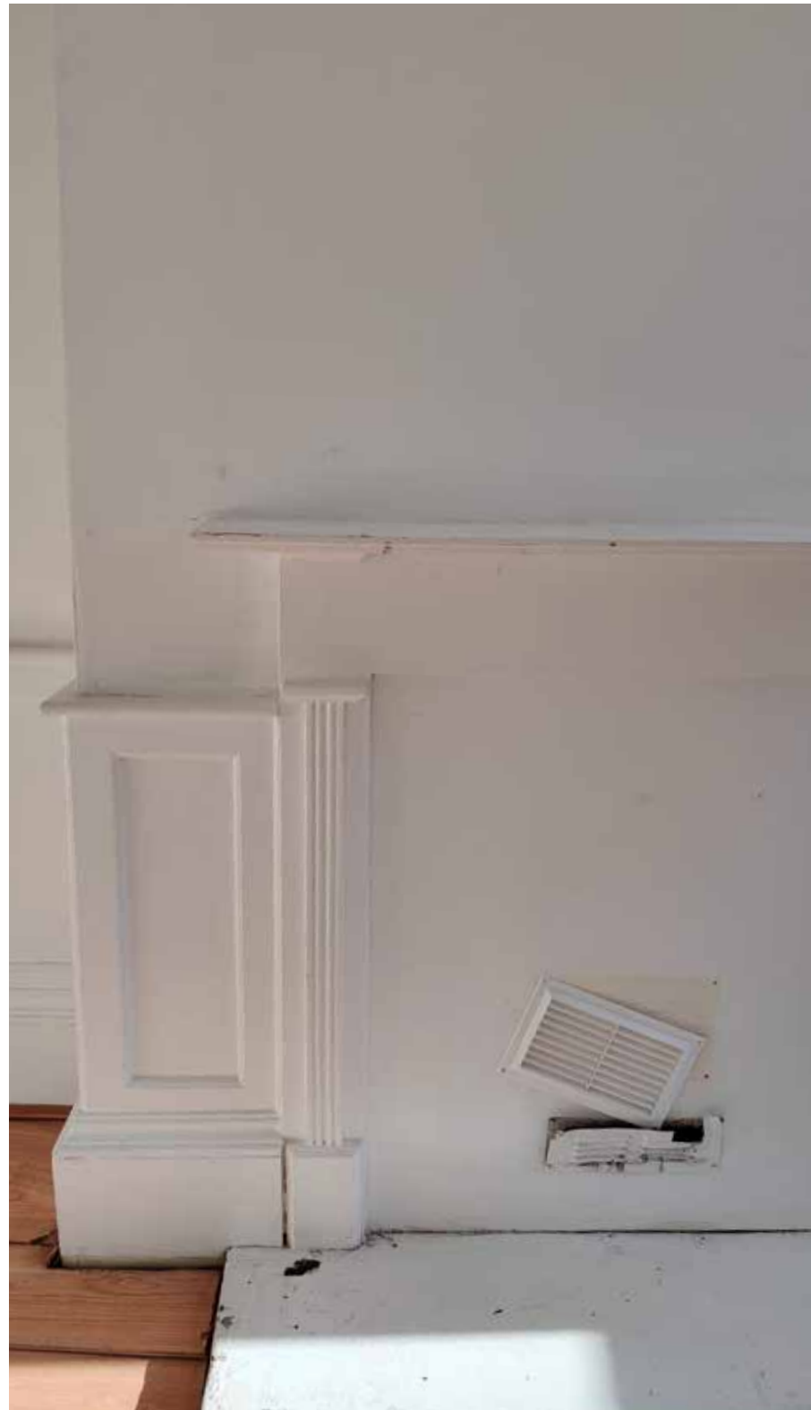
FIGURE 14. Existing Fireplace, Dado, Skirting and Panelling
