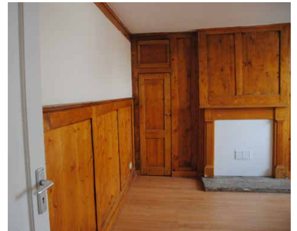
FIGURE 36. Existing Dado railing and Fireplace Detail
