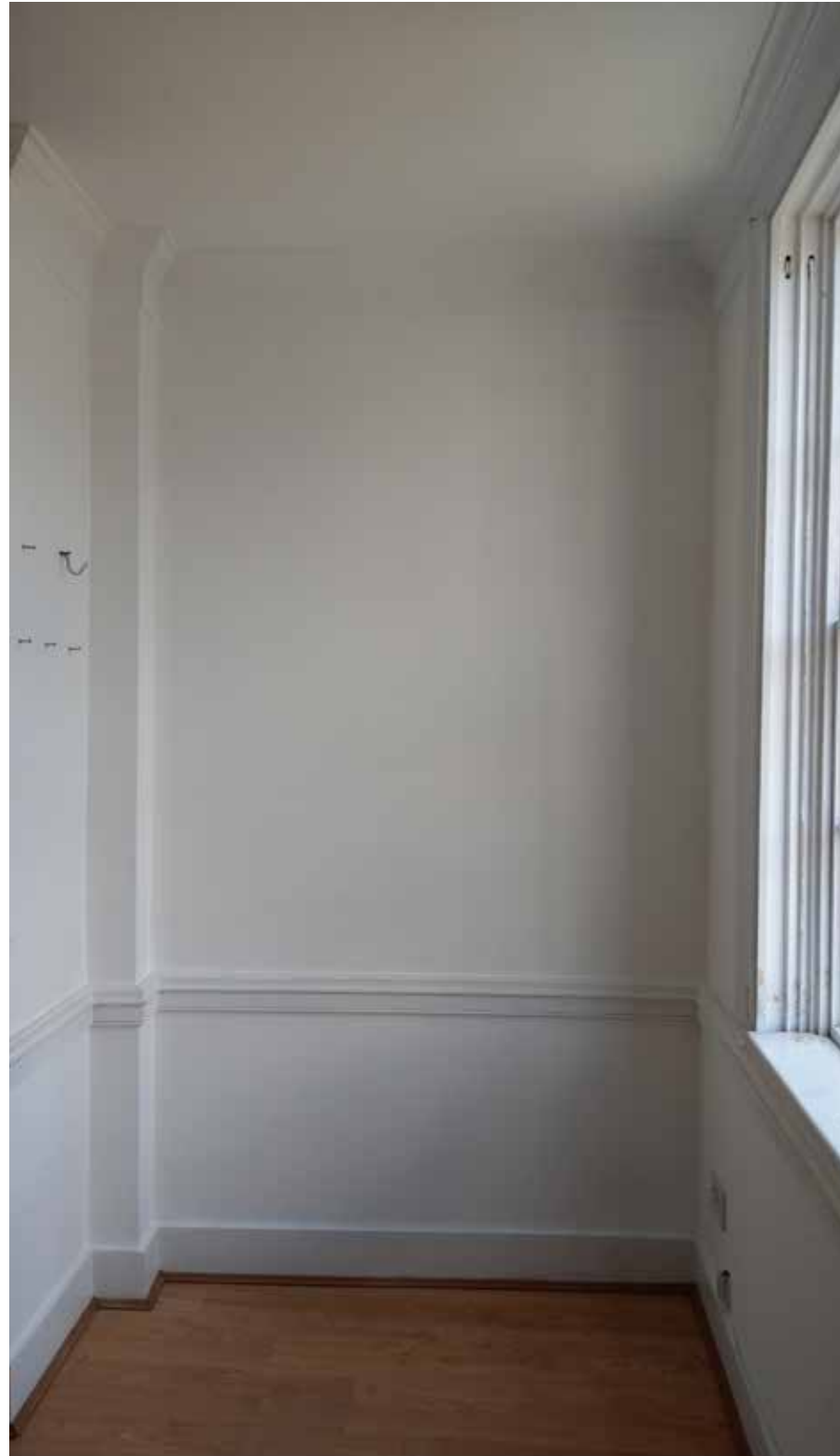
FIGURE 31. Existing Dado and Ceiling Cornice
