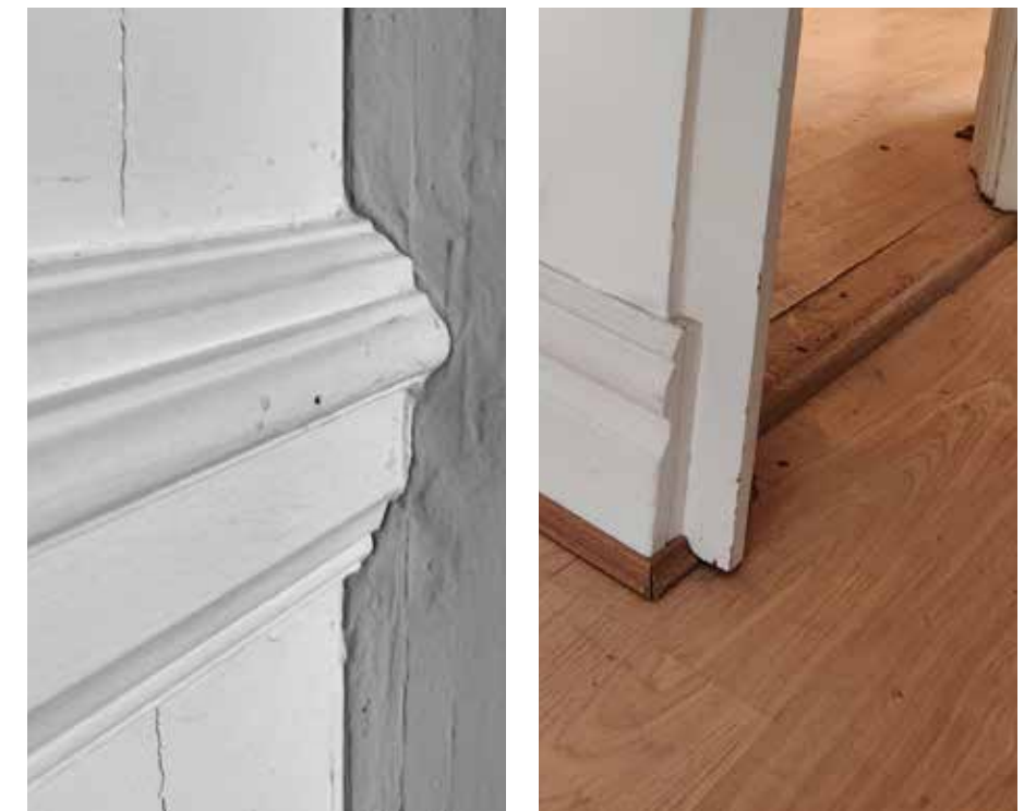
FIGURE 26. Existing Dado and Skirting Detail
