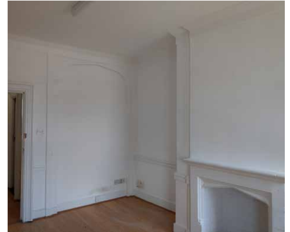
FIGURE 32. Existing Fireplace, Dado and Ceiling Cornice
