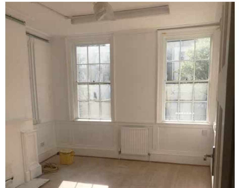
FIGURE 16. Existing Panelling and Ceiling Cornice
