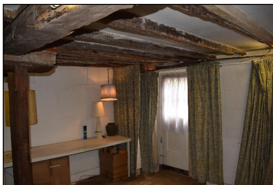
Photo 13: Ground floor timbers visible in the basement
