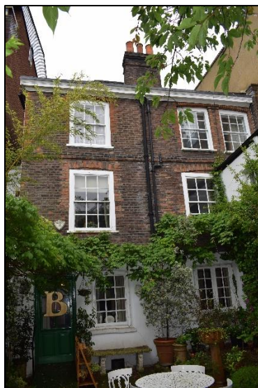
Photo 2: The rear elevation from the garden
