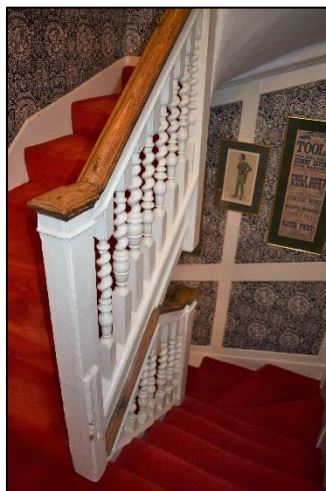
Photo 8: The staircase at first floor level
