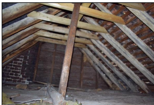
Photo 12: Part of the roof structure
