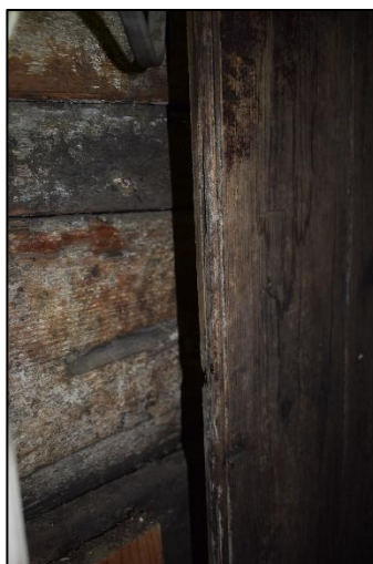
Photo 7: Possible original oak timber panelling behind later panelling in the kitchen
