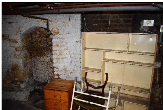
Photo 14: Base of the chimney and blocked doorway (behind the built-in shelves, right) in the rear basement
