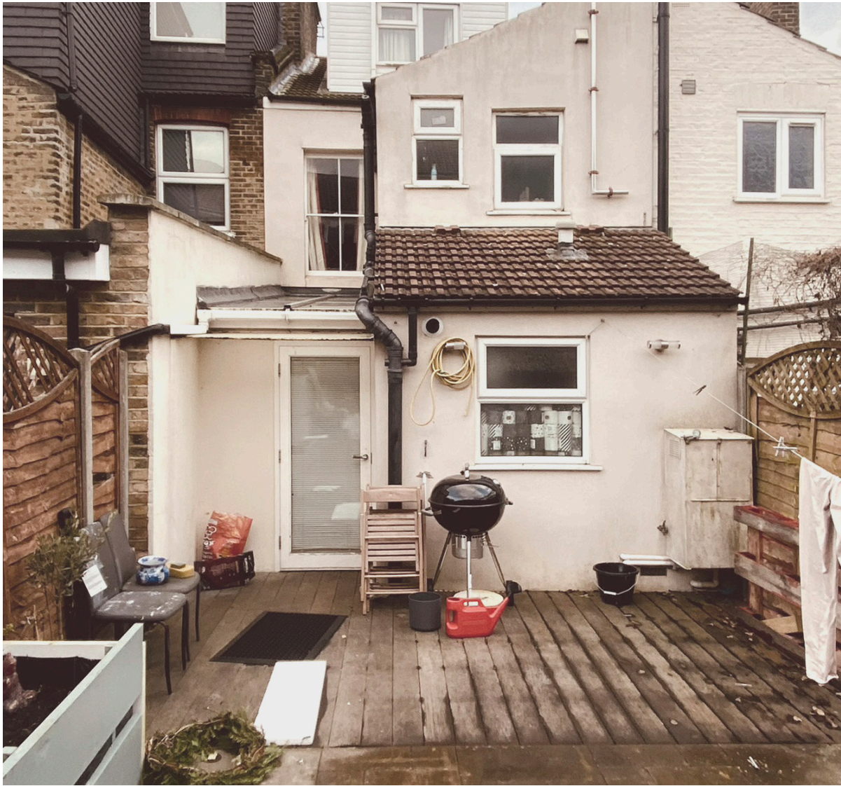
REAR PHOTO AS EXISTING
