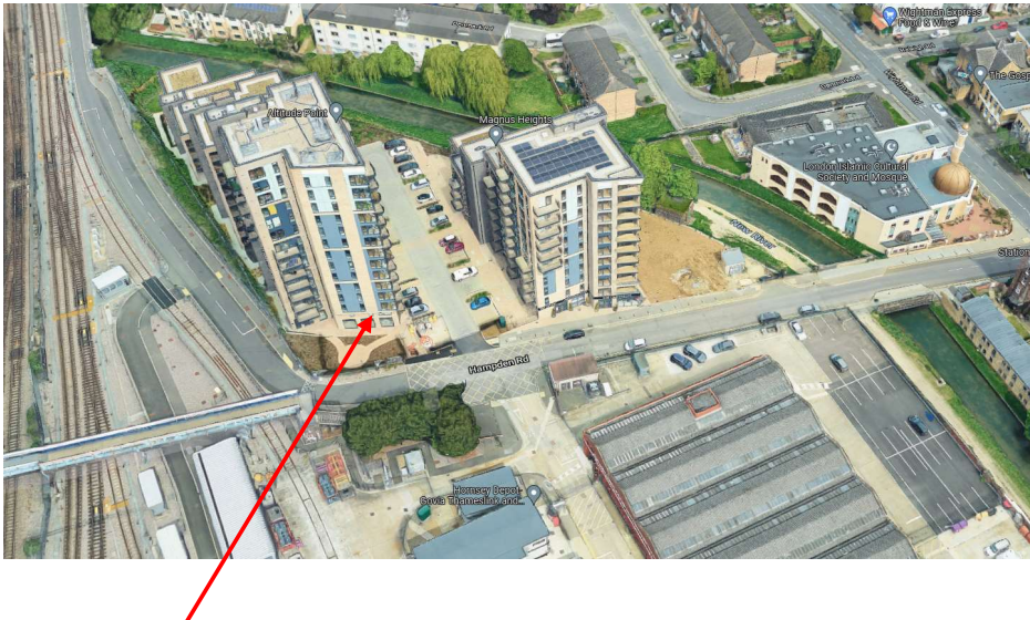
The application site
