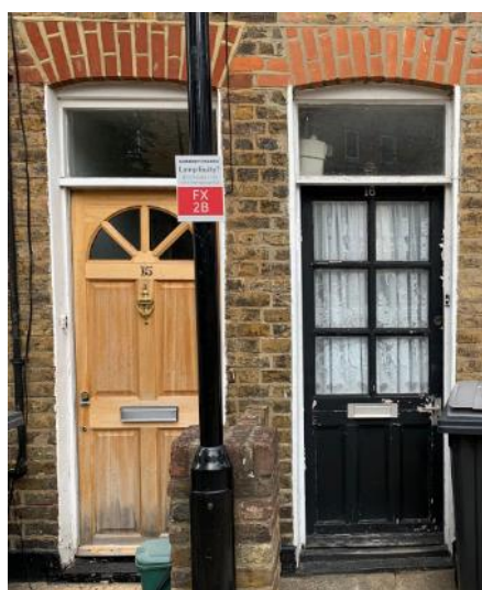
Figure 3: No.15 & 16 Front Entrance Doors
