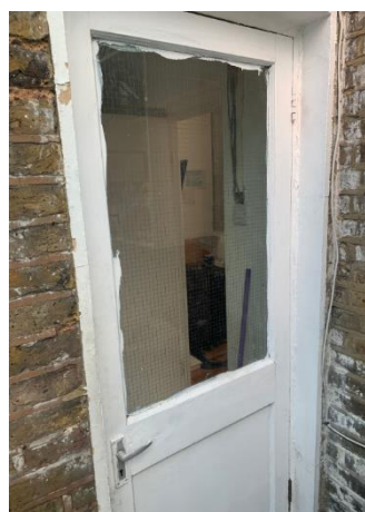
Figure 5: Rear External Door
