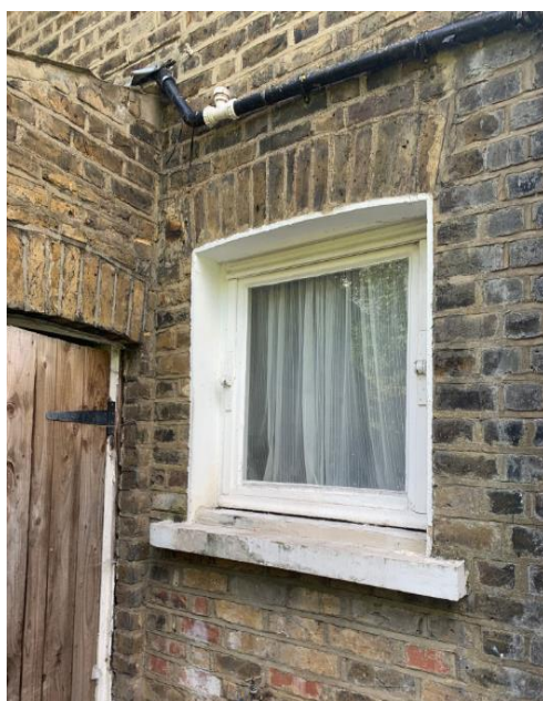
Figure 2: Front and Side Elevations
