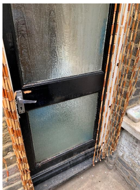
Figure 4: Rear External Door
