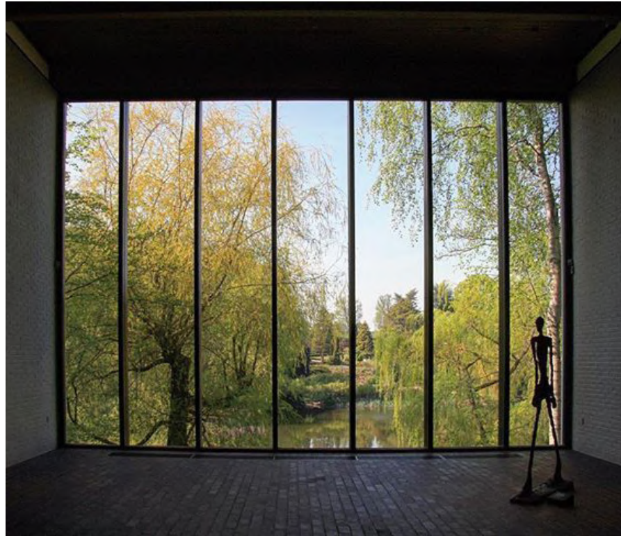
Timber window mullions defining views into landscape. Louisiana Museum of Modern Art by Vilhelm Wohlert and Jørgen Bo, Denmark.
