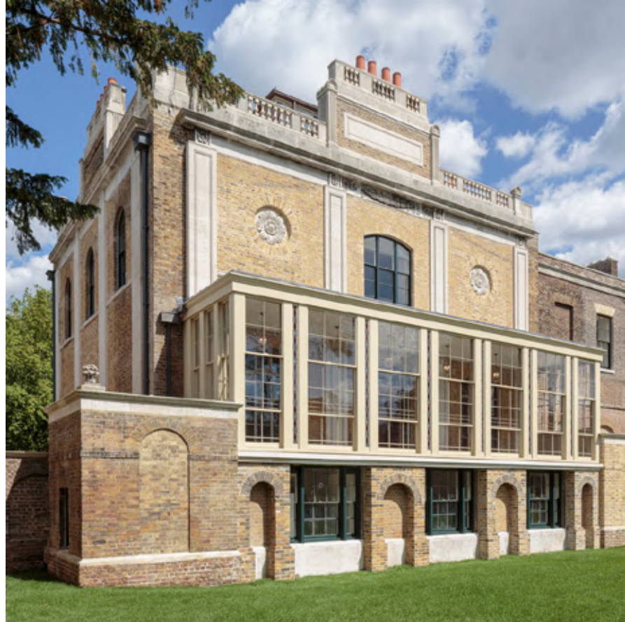
Historic glazed addition to English country house. Pitzhanger Manor House by Sir John Soane
