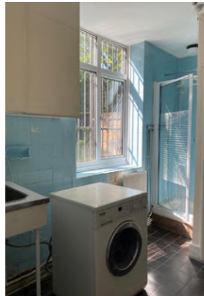
4. Existing kitchen condition
