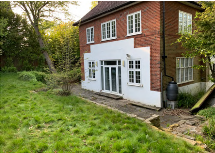
1. South facing side of Beaulieu House
