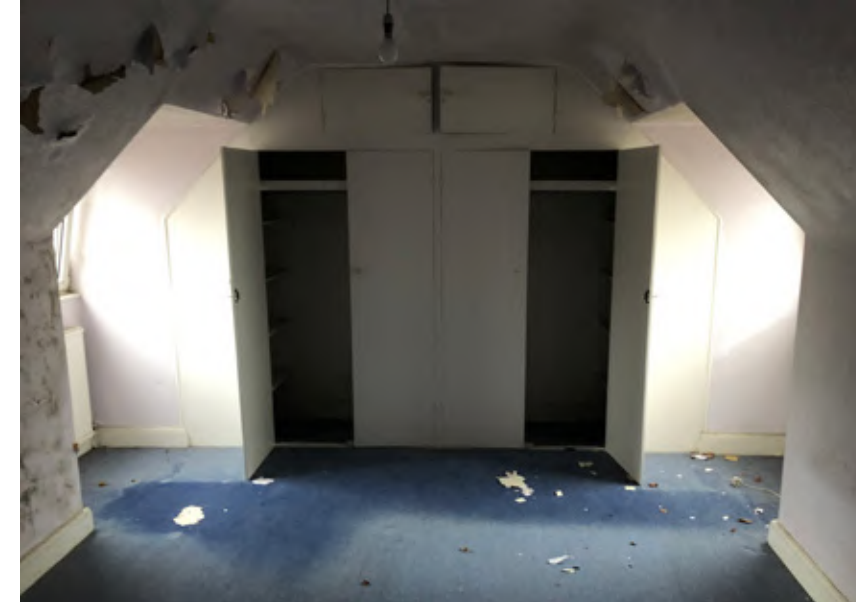
2. Existing roof space condition
