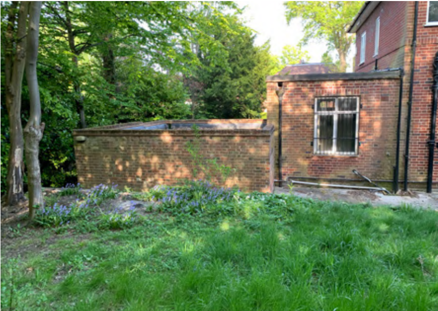
3. Rear view of the garage and secondary access porch
