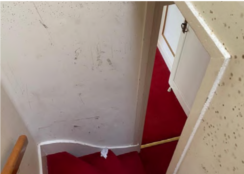
3. Existing Stairway condition
