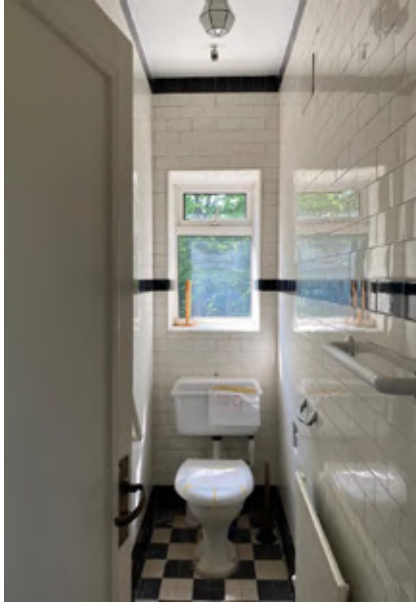
1. Existing W/C conditions
