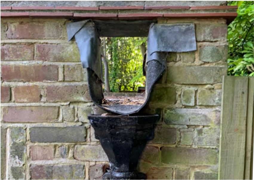
3. Gutter detail on garage extension
