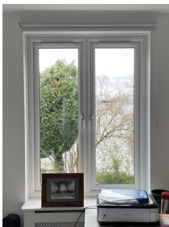
(Fig. 06) Window 01 Internal View.
