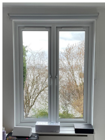
(Fig. 07) Window 02 Internal View.
