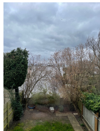
(Fig. 08) Window 02 External View.
