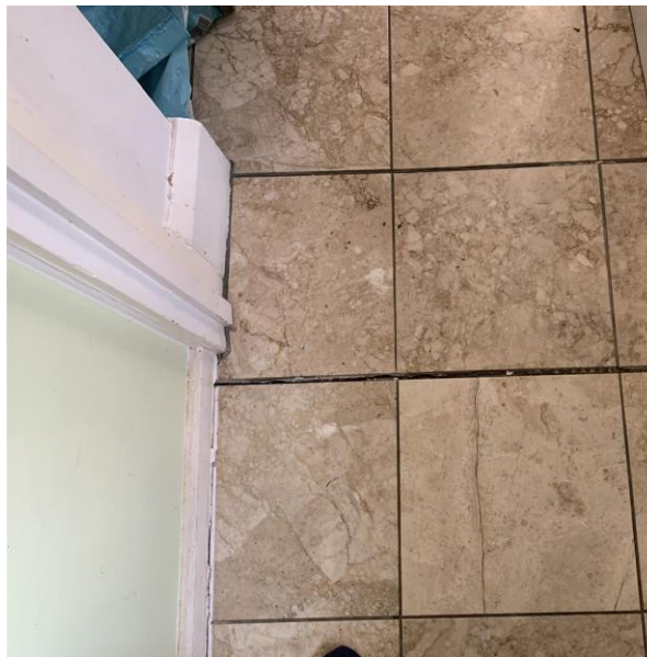
Utility Room Floor
