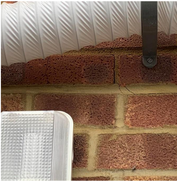
Above toilet window on rear wall
