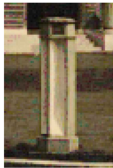
12 Archive photograph of original lighting bollard
