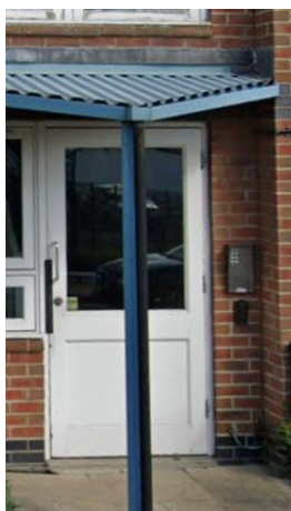
Figure 1: Existing Block entrance door
