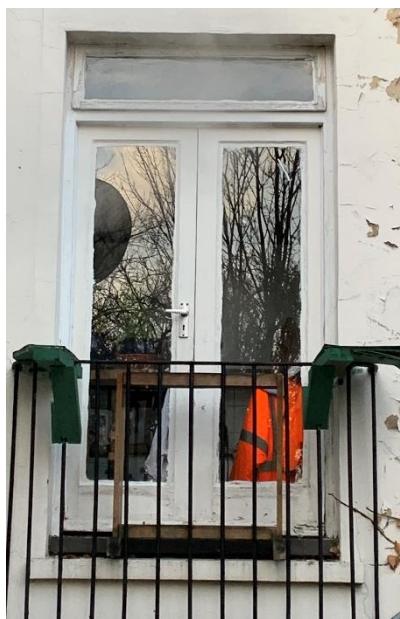
Figure 4: Existing rear doors
