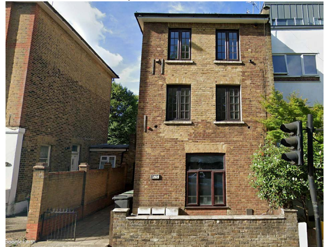
Front View of Flat 1 - 415 Archway Road
