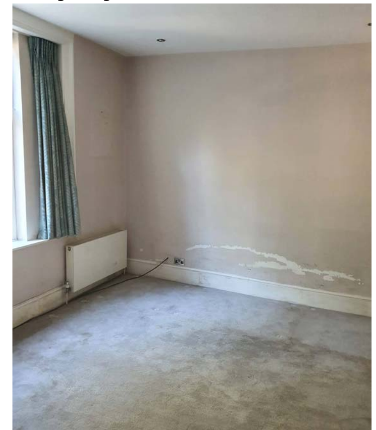
Existing Living Room
