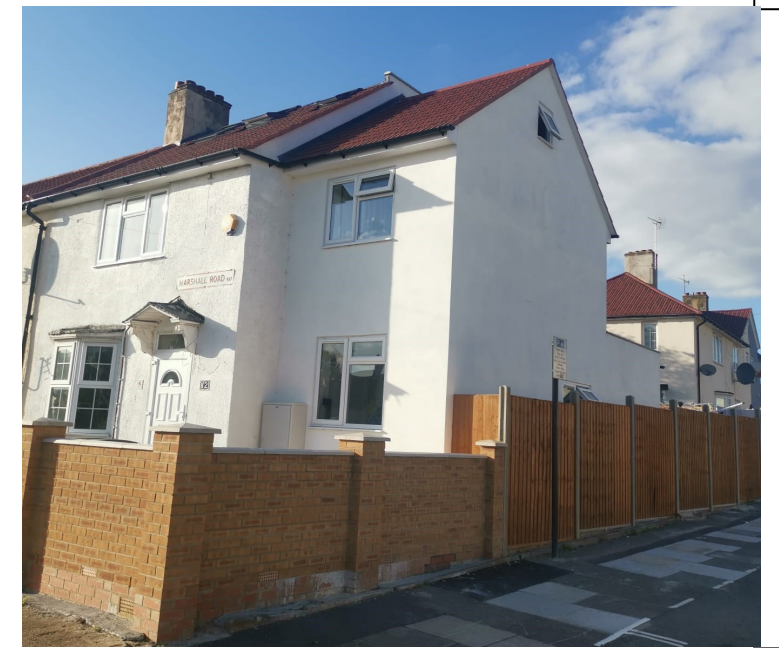
Photo 03—Front of neighbouring properties with similar loft conversion (2 Marshall Road N17 7AP)
