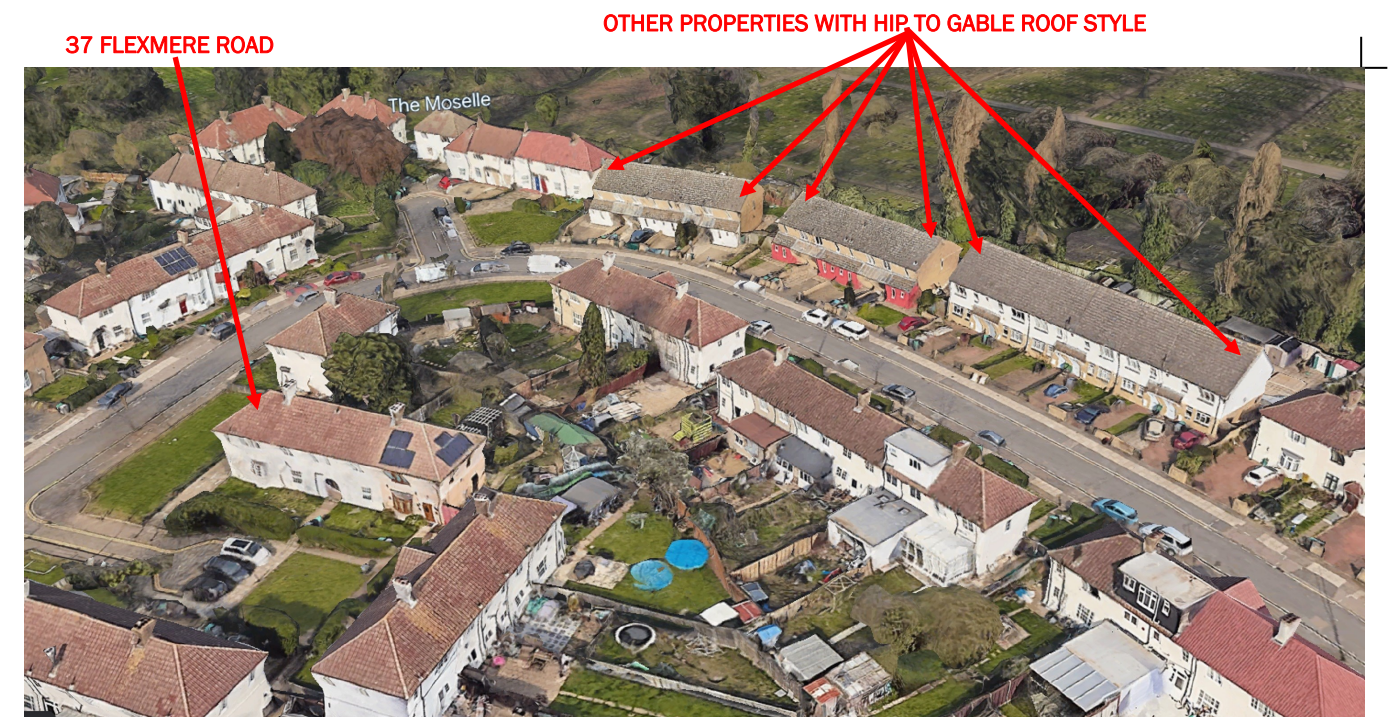
Photo 05—Application site and neighbouring properties with hip to gable roof style
