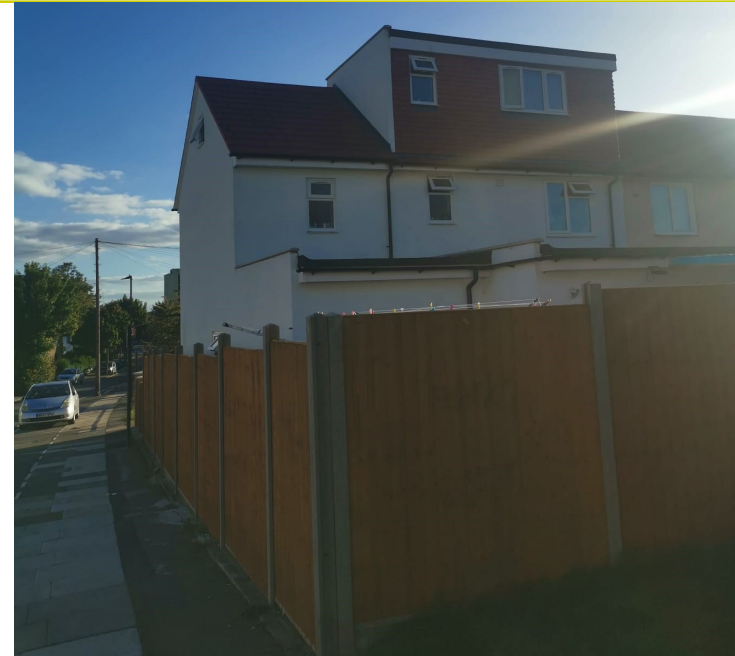
Photo 02—Rear of neighbouring properties with similar loft conversion (2 Marshall Road N17 7AP)
