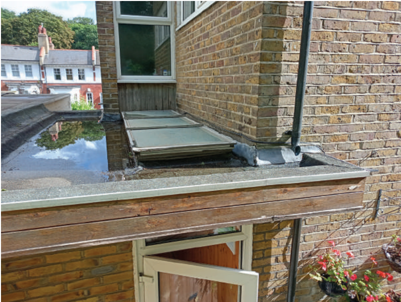
Rear view of the property - existing extension & roof light
