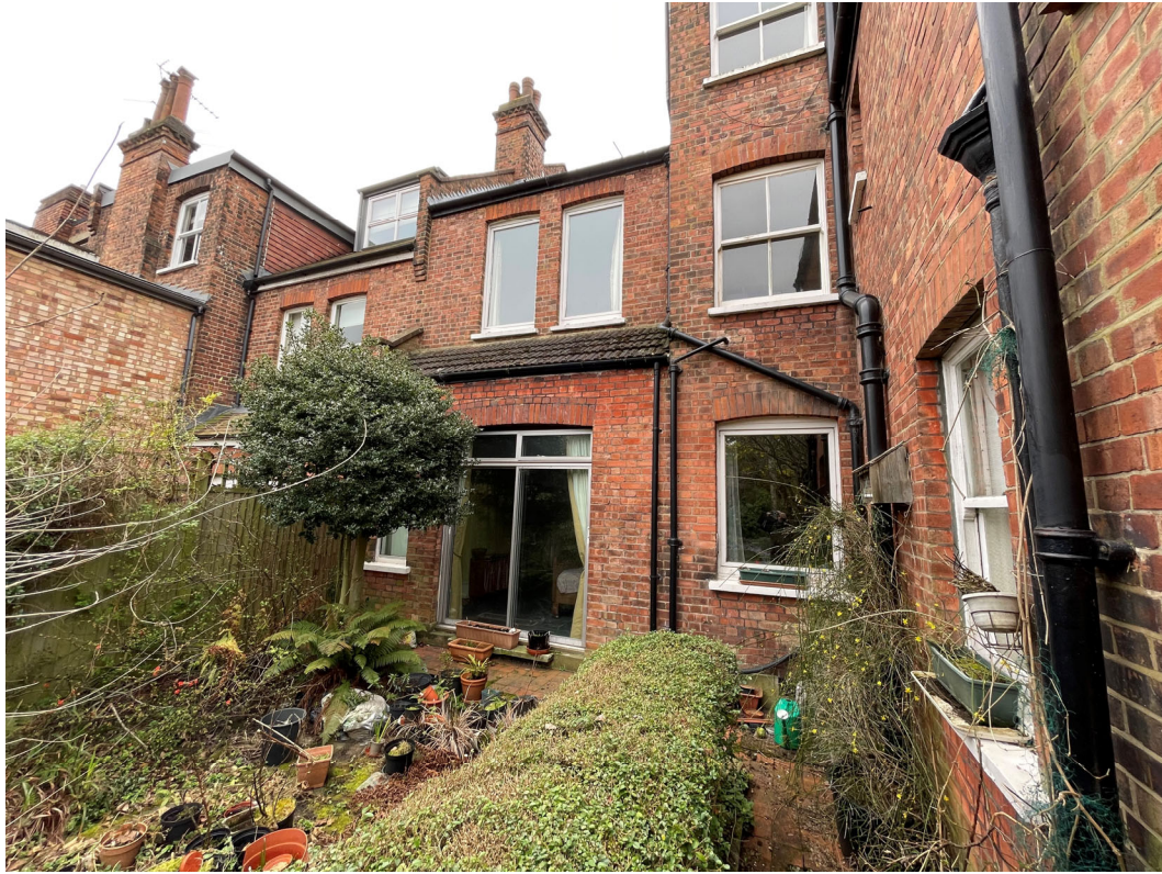
View of the rear / side boundary
