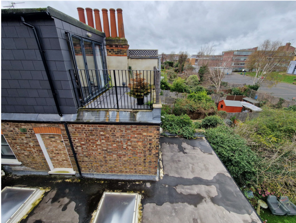
View of flat roof where access stair would be located
