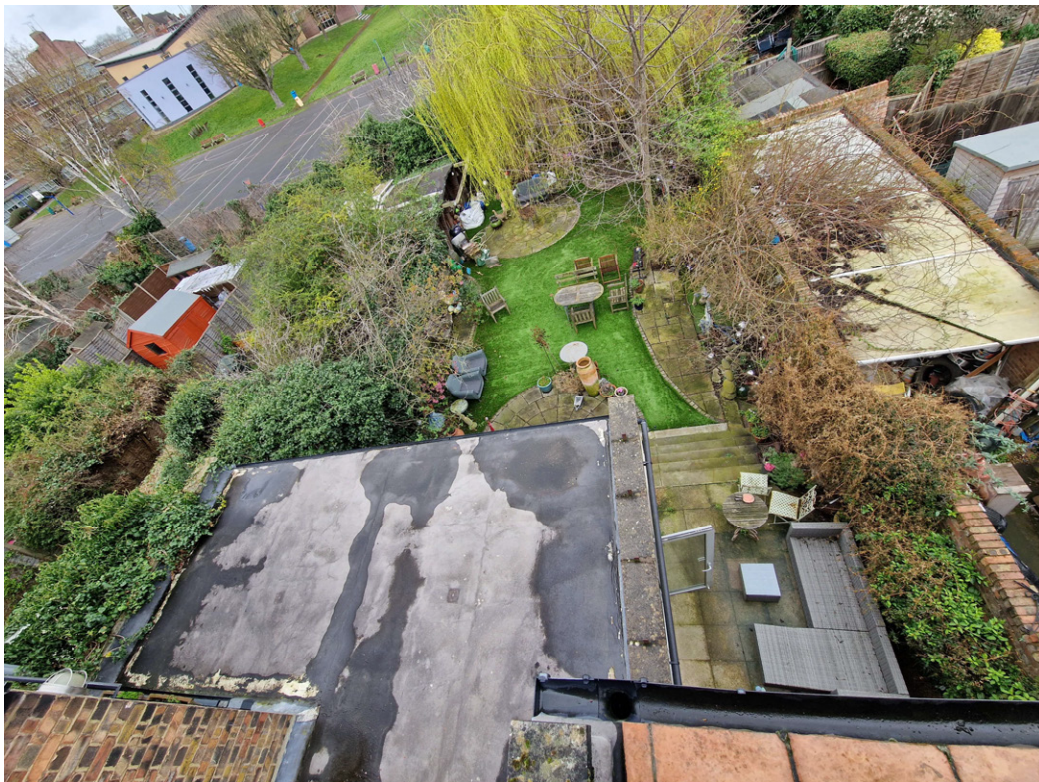
View of flat roof and garden
