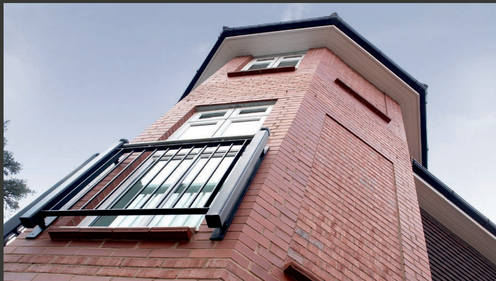
Apartments, Streetly, West Midlands Ravenhead Smooth Red & Chester Red Blend - AN.2.5 External Angle
