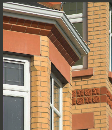
Private Housing, Douglas, Isle of Man Cheddar Golden & Cheddar Red - PL.2.1 Plinth Header, I.PL.15.1 Wide Bed Plinth Stretcher & PL.8.9 Plinth External Angle
