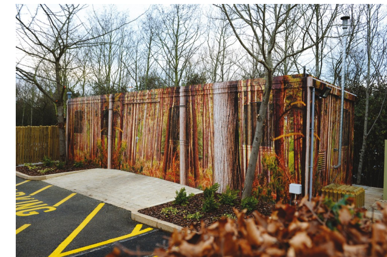
The Portacabins will be finished with a Vinyl wrap in Hale Village colour scheme
