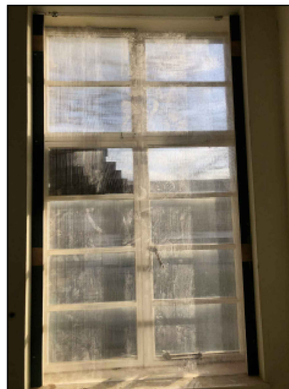
04 SITE EXISTING WINDOW PHOTOGRAPH
