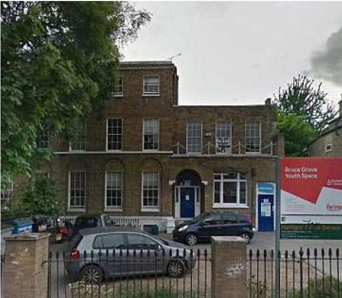
Front access to No.10 Bruce Grove
