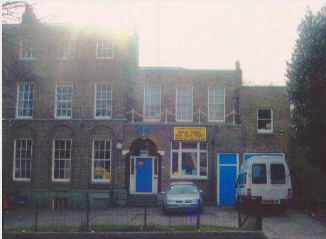
No. 10 Bruce Grove prior to demolition of North wing, 2004
