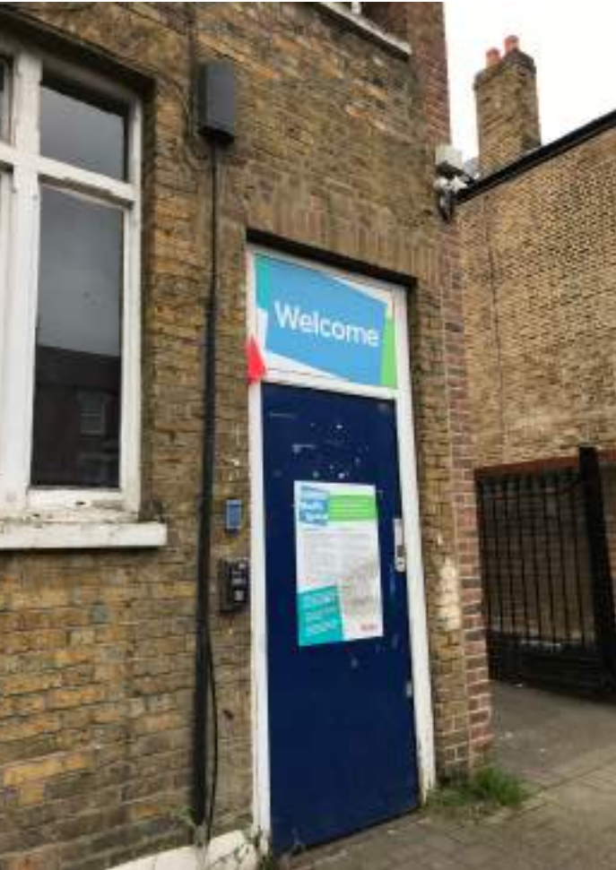
Front access to No.10 Bruce Grove
