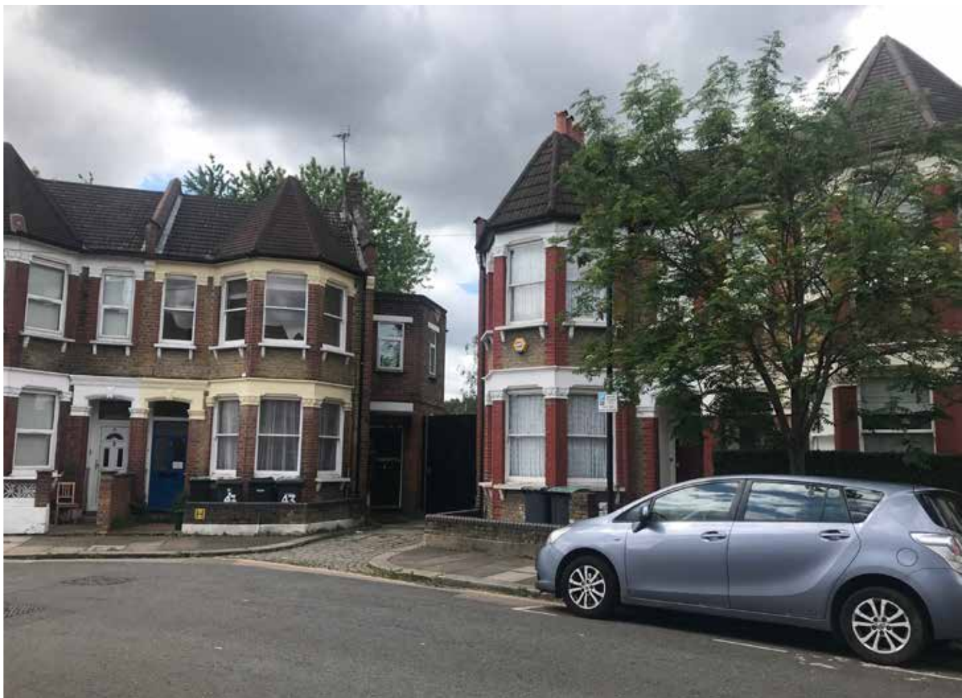
View of site entrance from Belmont Avenue
