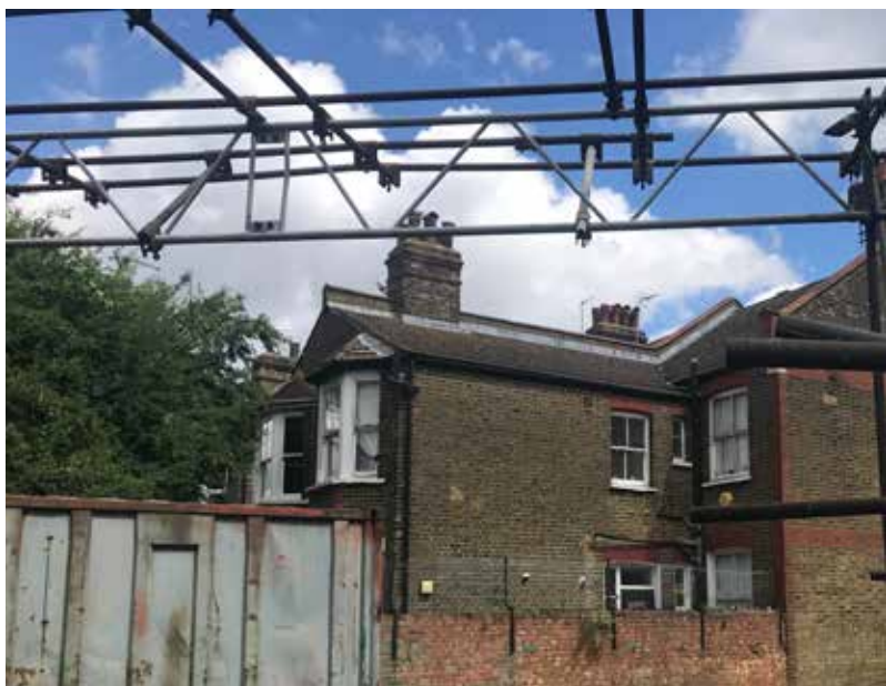
View to North of site showing neighbouring terrace. Note: brick garden wall and chamfered bays. Scaffolding shown above
