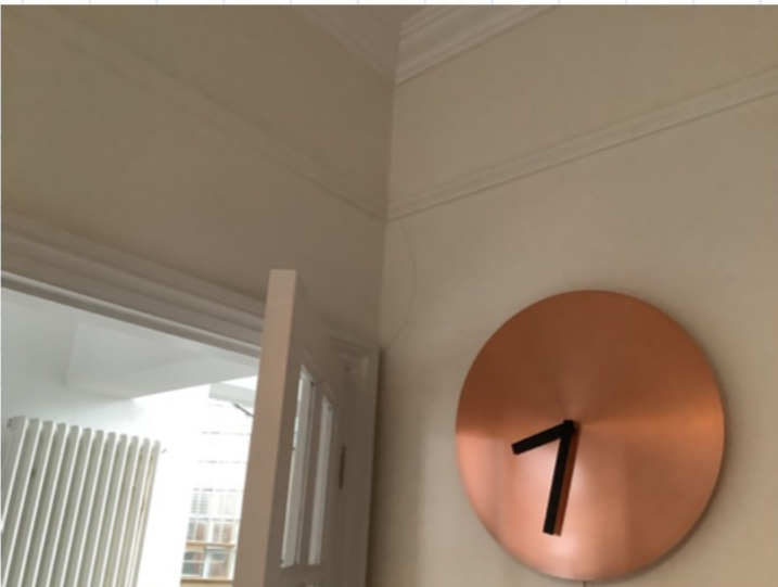
Wall crack to lounge
