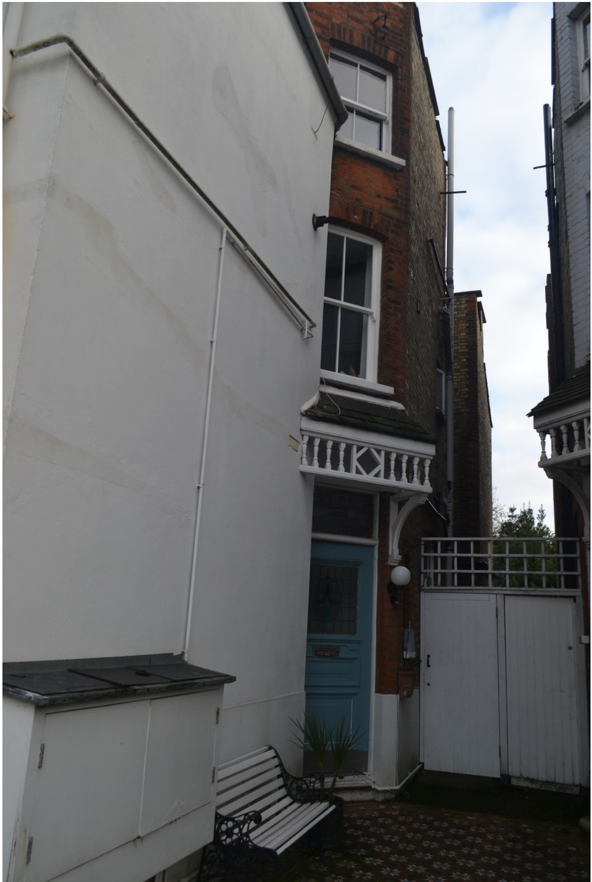
Photograph 4 – Main entrance to side.
