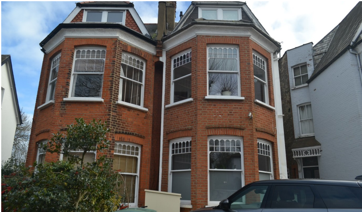
Photograph 2– Photograph 3 – Right hand property and front elevation no change.
