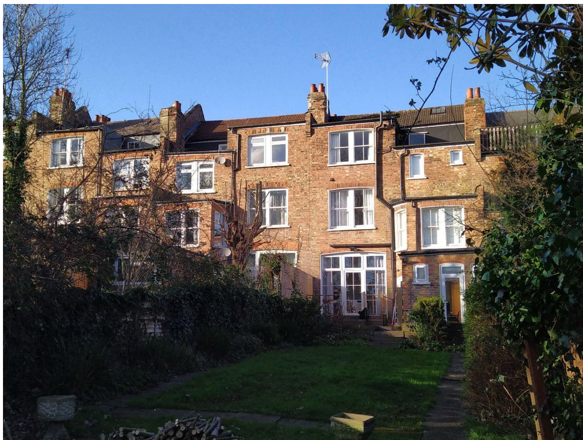
Current View of the Rear Elevation
