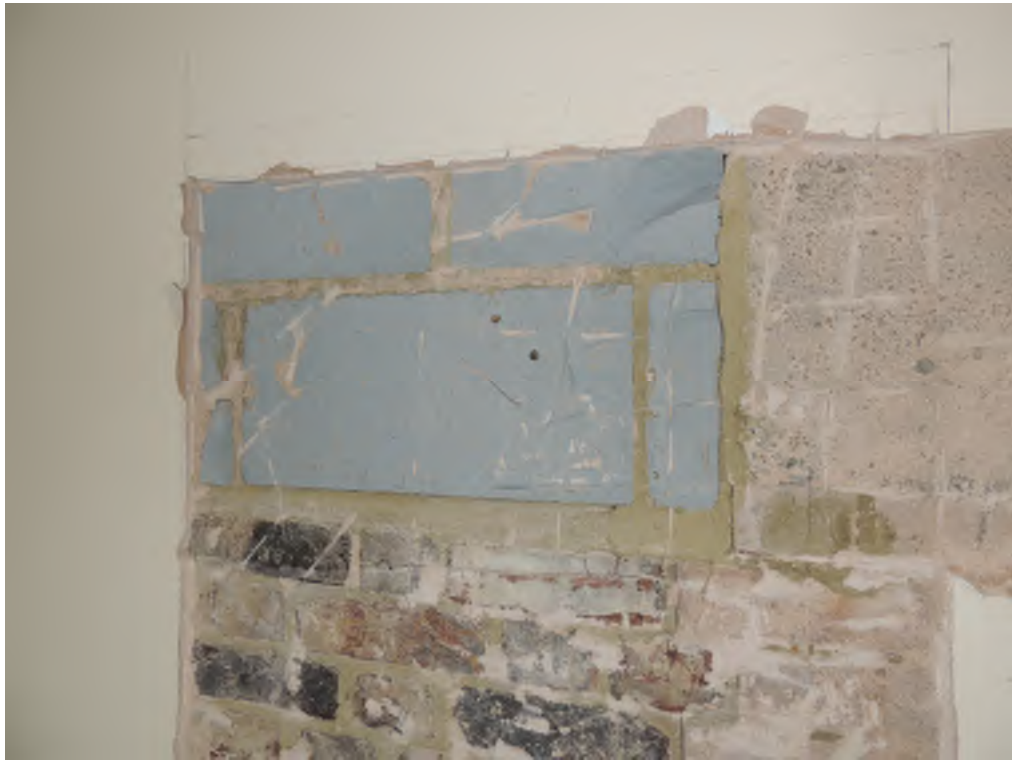
Photograph 3: Removed finishes at proposed doorway
