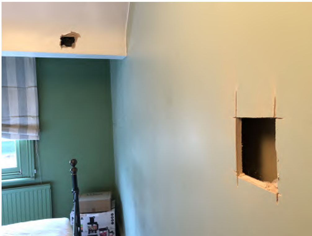
Photograph 9: Removed finishes at middle of existing wall
