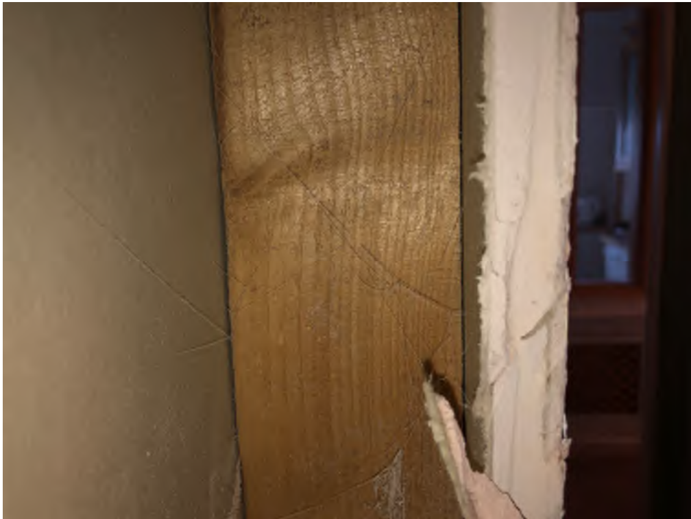
Photograph 10: Removed finishes at middle of existing wall
