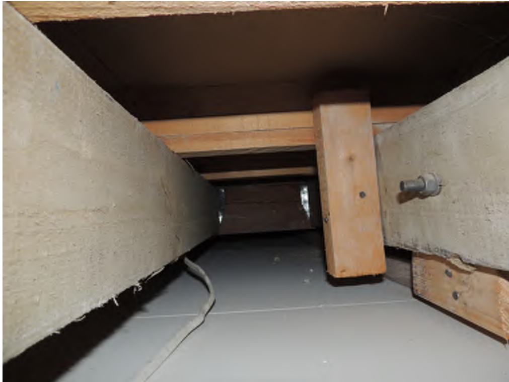
Photograph 6: Floor structure at foot of proposed doorway
