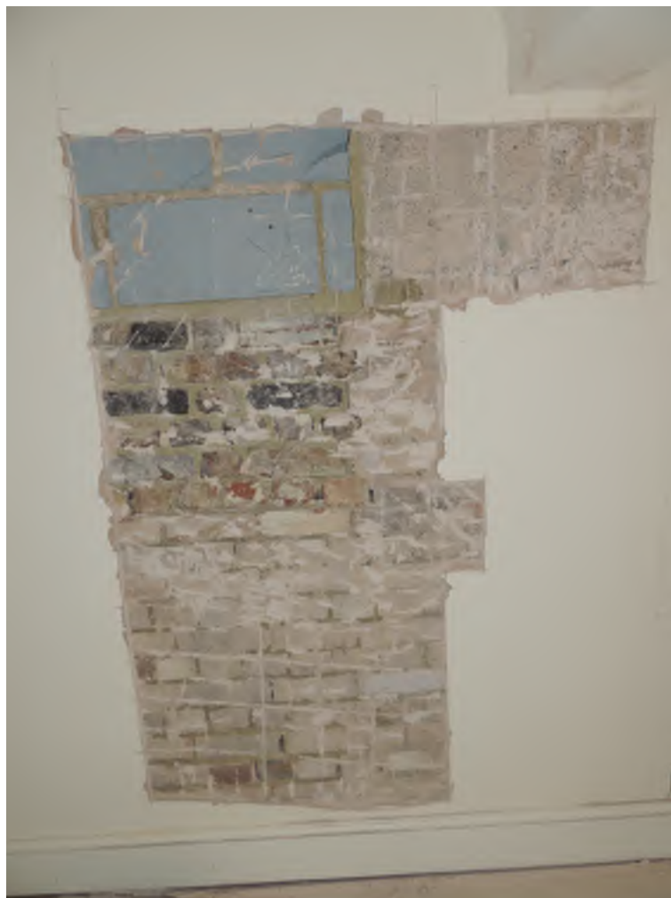
Photograph 2: Removed finishes at proposed doorway
