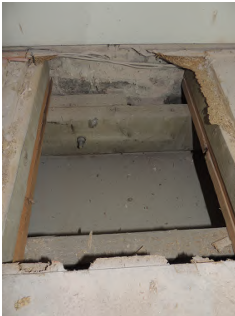
Photograph 5: Floor and wall structure at foot of proposed doorway
