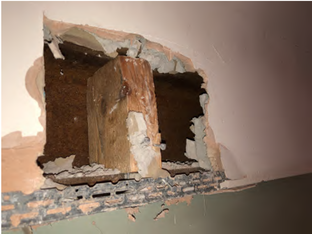
Photograph 7: Removed finishes at head of proposed doorway
