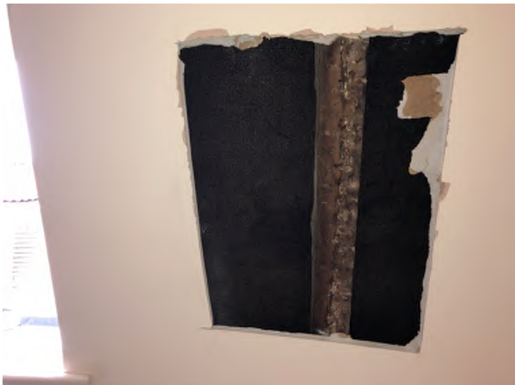
Photograph 14: Removed finishes at proposed dormer window
