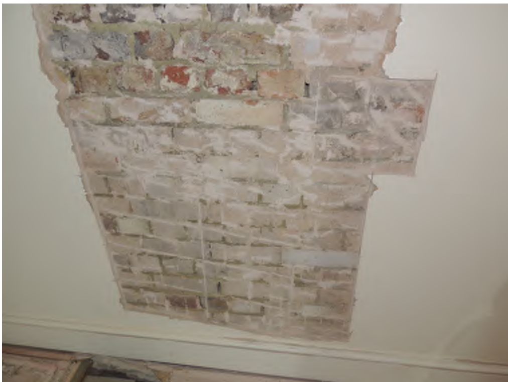
Photograph 4: Removed finishes at proposed doorway
