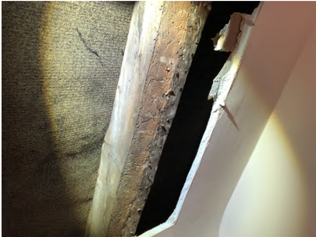
Photograph 15: Removed finishes at proposed dormer window
