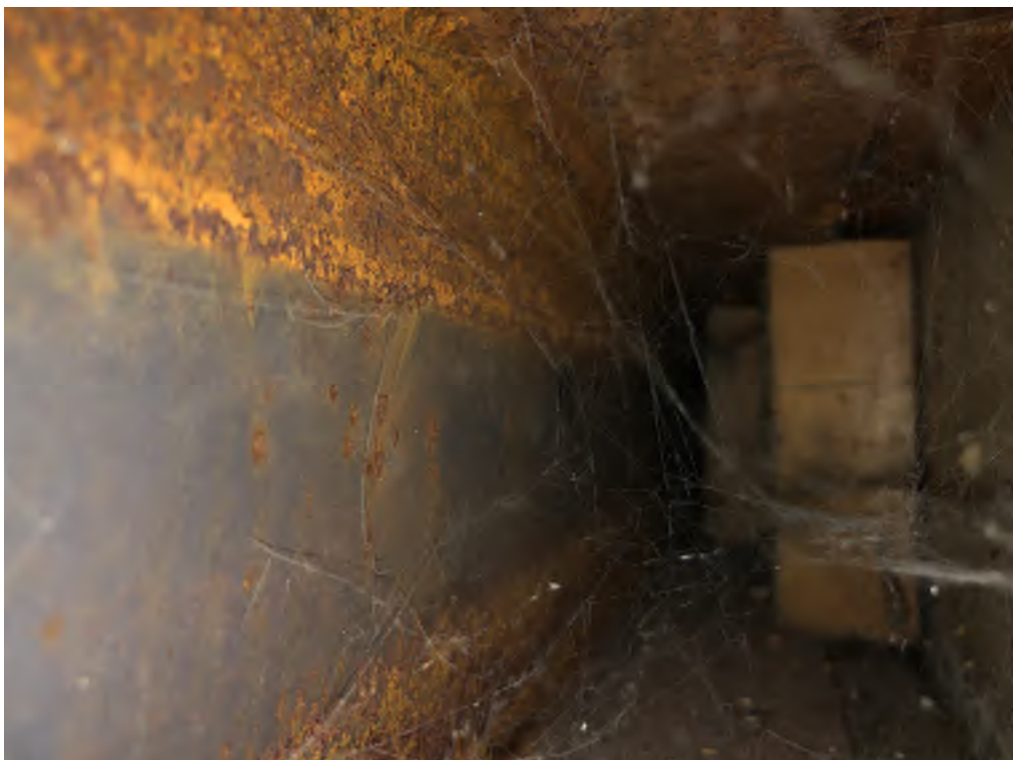
Photograph 8: Removed finishes at head of proposed doorway
