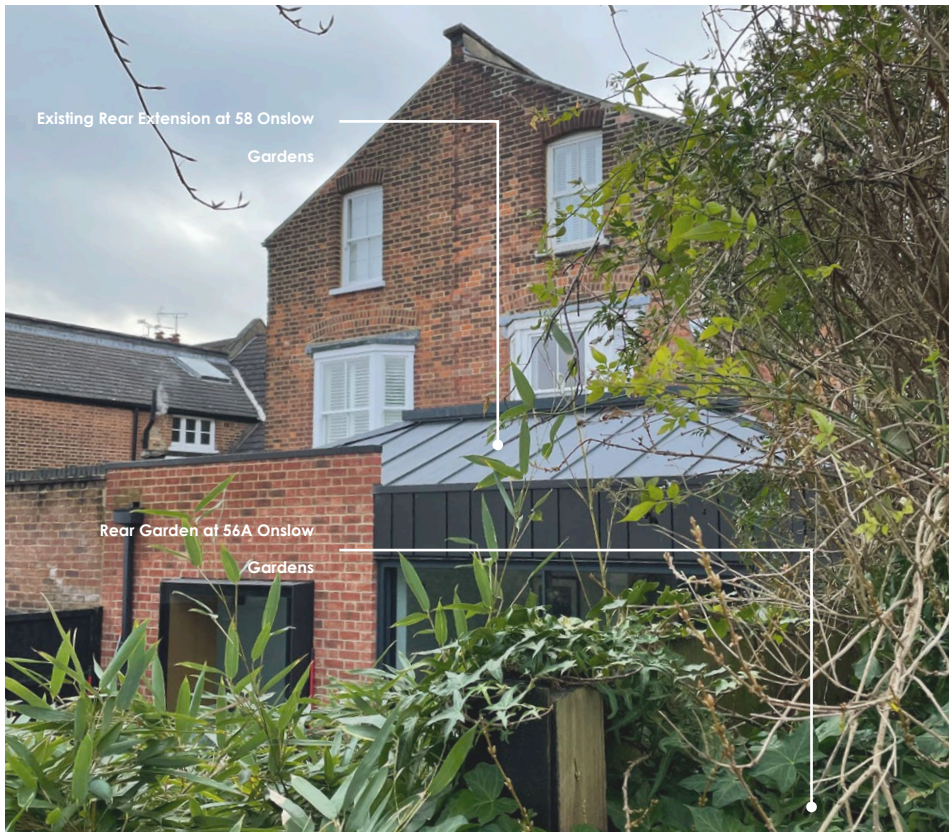
4. Existing neighbouring rear extension at 58 Onslow Gardens
