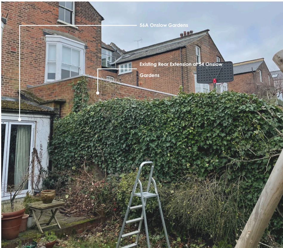
3. Existing neighbouring rear extension at 54 Onslow Gardens
