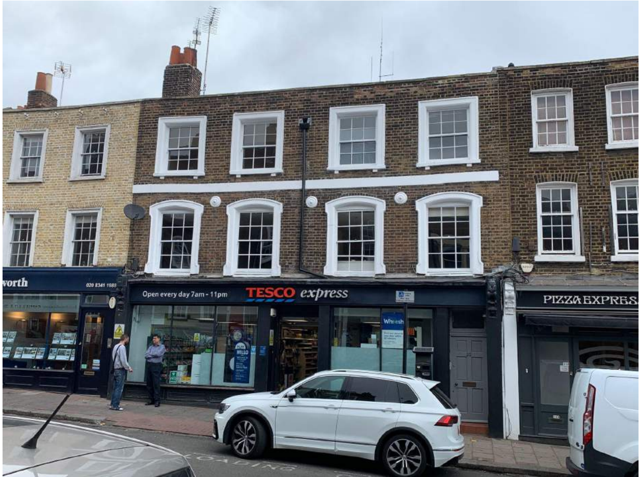
Front of Flat C (second floor windows) 32-34 Highgate High Street.
