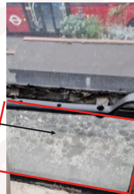
View of ledge through lower windows.
