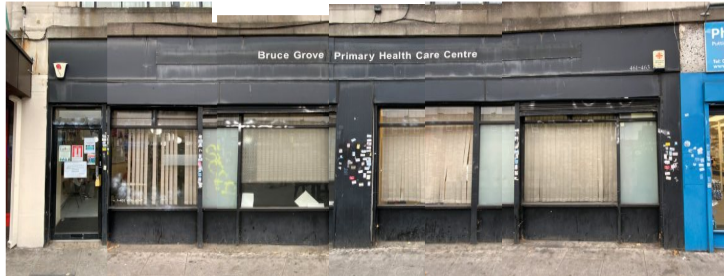
It is proposed that the shopfront is refurbished, with repainting of the frames and panels to the pilasters in black as existing
