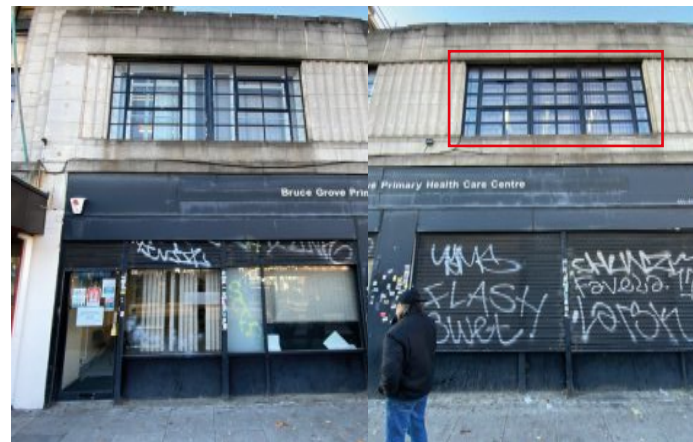
The south window (left) is original but in poor condition and has reached the end of its useful life. It is proposed to be replaced with a new steel-framed double glazed window to the same design as the north window (right).
