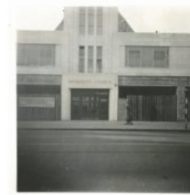
ORIGINAL ENTRANCE - SIMPLE & UNDERSTATED - SIMPLE TYPEFACE 'METHODIST CHURCH'
