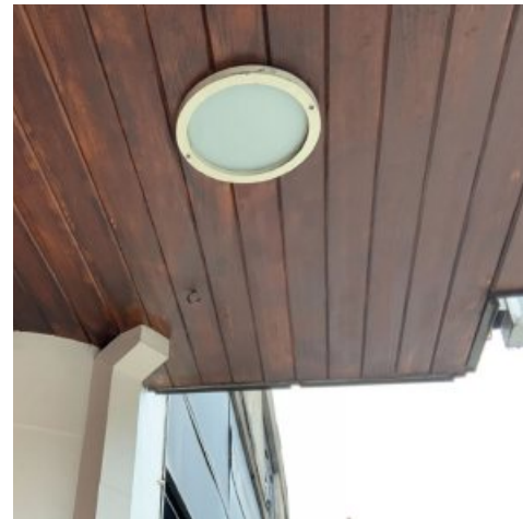
Underside of canopy with timber boarding; this could be retained with the boarding re-finished.
