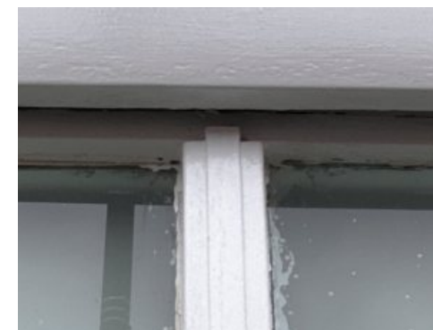
Original awning bracket and Art Deco styled moulding to mullion
