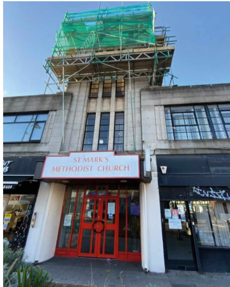
The existing entrance screen is a modern replacement in aluminium with red decorations. This is at odds with the Art Deco styling of the wider façade and has a negative impact on the building as a whole.
