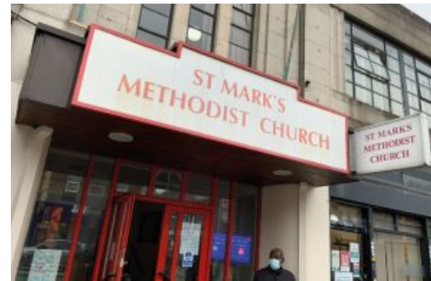
Front view of canopy with projecting sign; both are detrimental to the Art Deco character of the building
