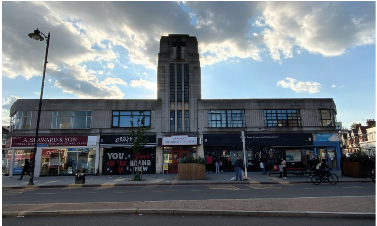
Signage varies in design between the shop units, resulting in visual disunity and impacting negatively on the symmetrical façade
