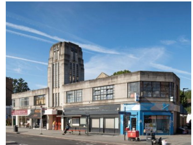
View of St. Mark's Methodist Church 'block' looking south
