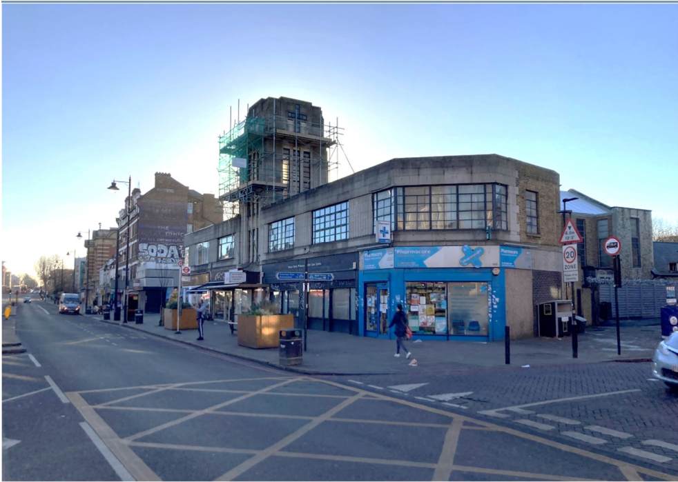
St Mark's Methodist Church (Viewing North and East Elevations)
