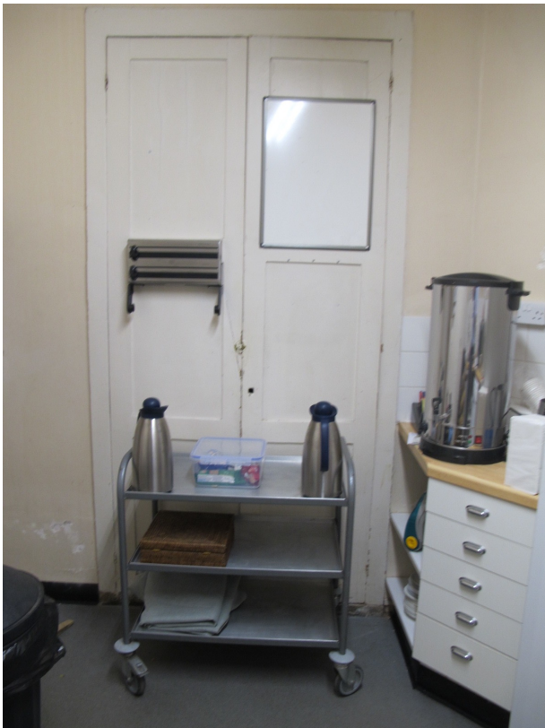
G2 - Joinery on East Wall
