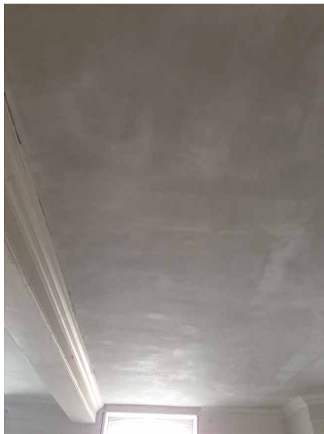
Photo 4 Completed repaired ceiling with skim coat finish made good
