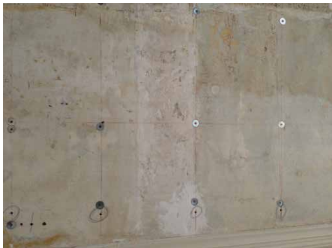
Photo 3 Grid of Screw and Washer fixing securing existing lime plaster ceiling
