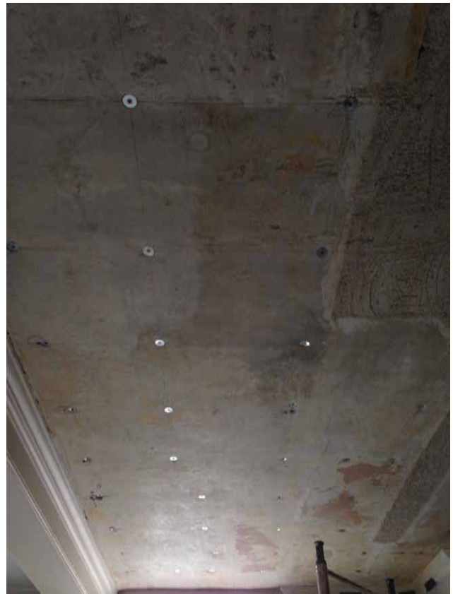
Photo 2 Ceiling secured with screws and washers
